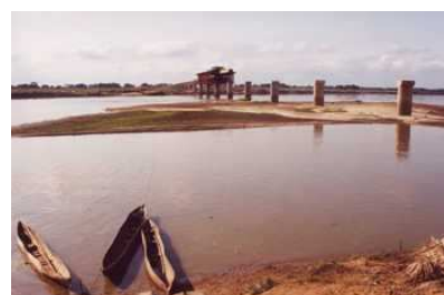
Rufiji River bridge under development, October 2001.
