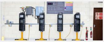
Explosive gases are given off when batteries are charged. The risk of an explosion is great if the gases are allowed to collect. When charging batteries, ensure you have a suitable Charging Station by following our guide.
