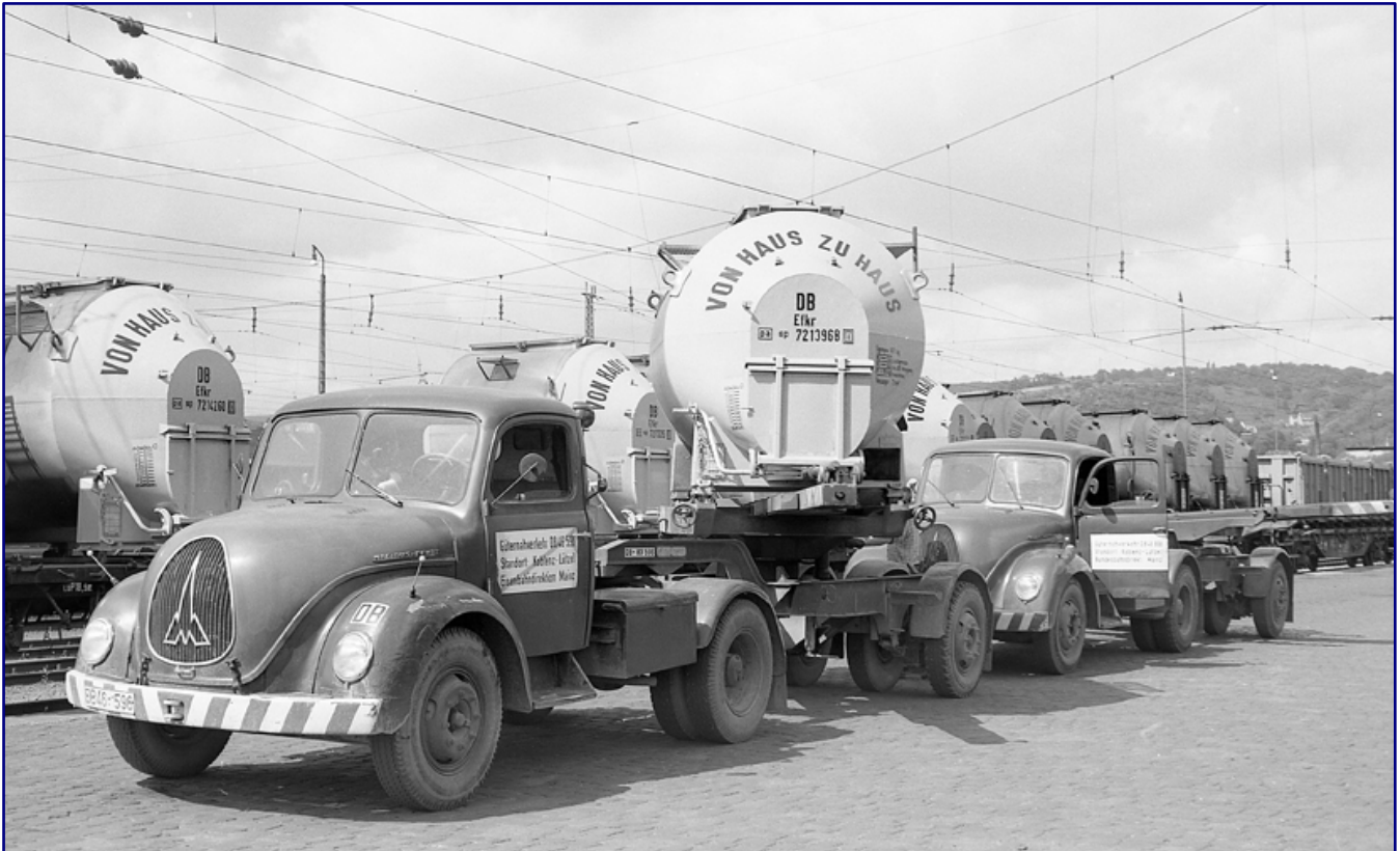
In August 1961, the loading of an Etkr container for fine bulk material by an Ackermann delivery vehicle was recorded in a sequence of pictures at the Koblenz-Ehrenbreitstein railway station. The vehicle with the registration number DB 49-596 drove parallel to the train on the loading road and swivelled the trailer 90 degrees over to the container wagon BTs 50. The Pa container is then rolled on rails onto the trailer and lashed there (top photo). Once it has been fixed securely for transport, the trailer swivels in again (bottom photo) and assumes its travel position. Photos: Sig. Eisenbahnstiftung
