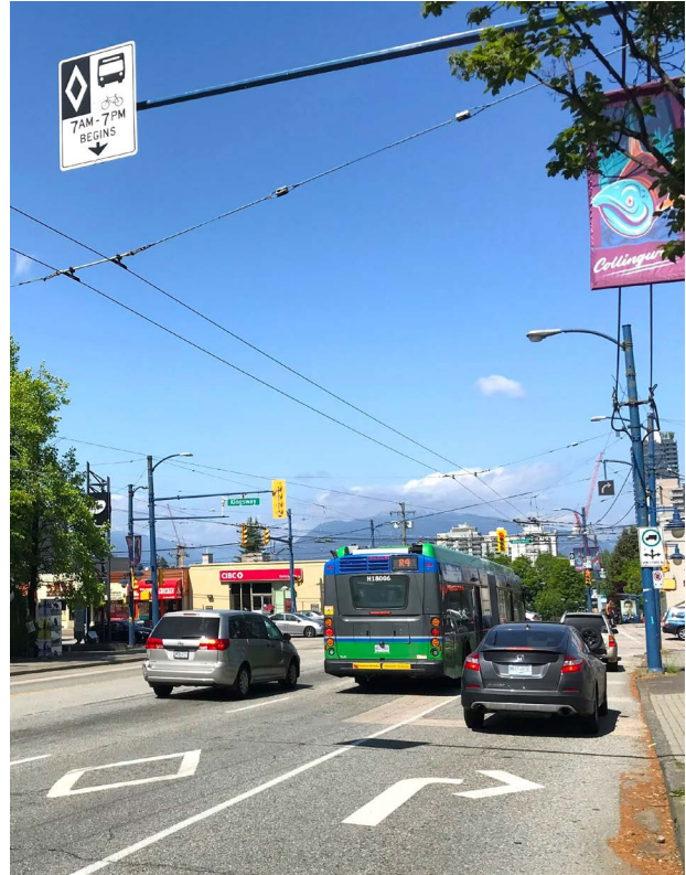
The approach lane on Joyce St at Kingsway is supported by a right-turn pocket. Parking was removed to lengthen this pocket and minimize friction with buses. The project reduced average travel times by more than 30% all day.
