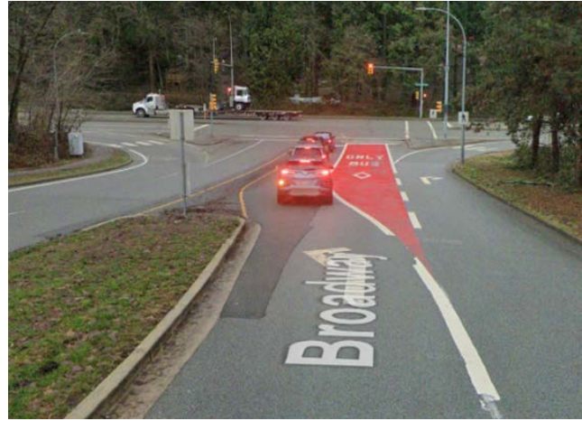
Before (left) and after (right) showing a bus queue jump lane with transit signal priority that was installed at the intersection of Broadway and Gagliardi Way in late 2020 (Google Street View).
