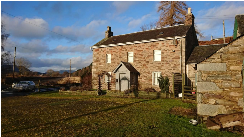
Photograph 14: The Range of Guay Farmhouse viewed from the west
