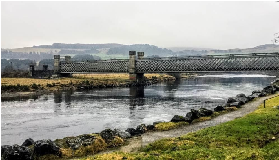
Logierait Railway Viaduct Over River Tay (Asset 753, Figure 15.1e)
