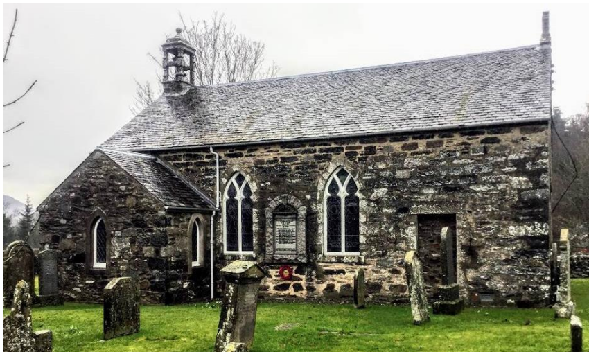
Photograph 17: Dowally Church (Asset 208)
