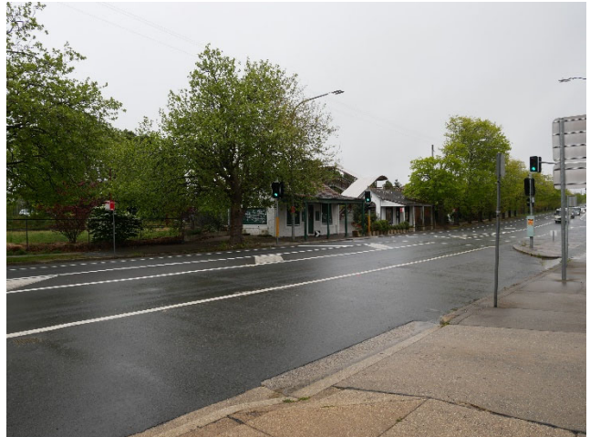
Figure 15 The pair of retail buildings on the Great Western from further south (Source: Purcell, 15 October 2021).
