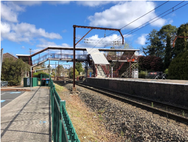
Figure 12 View south from the Great Western Highway Carpark to the footbridge and level crossing. (Source: Purcell, 22 September 2021).
