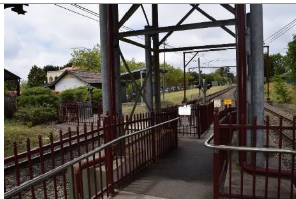
Figure 72 View of the level crossing ramp to the platform
