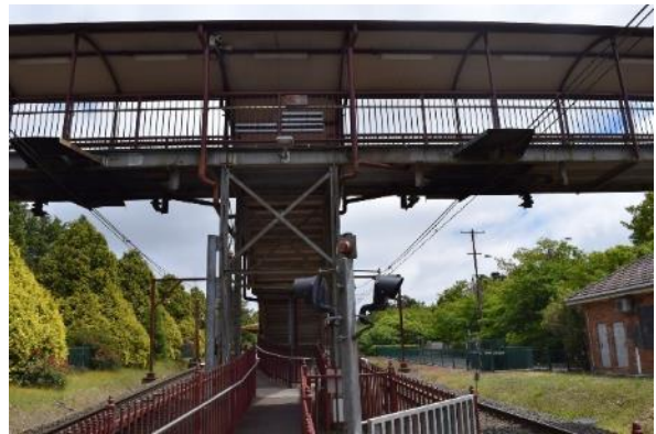
Figure 82 View of the footbridge from the level crossing
