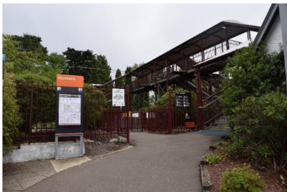
Figure 69 Entrance to the level crossing from the Great Western Highway
