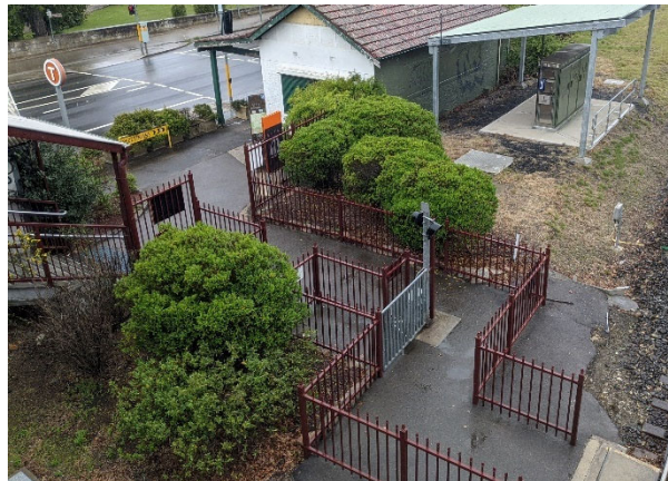
Figure 29: Existing picket style fencing. Source: Purcell, October 2021.
