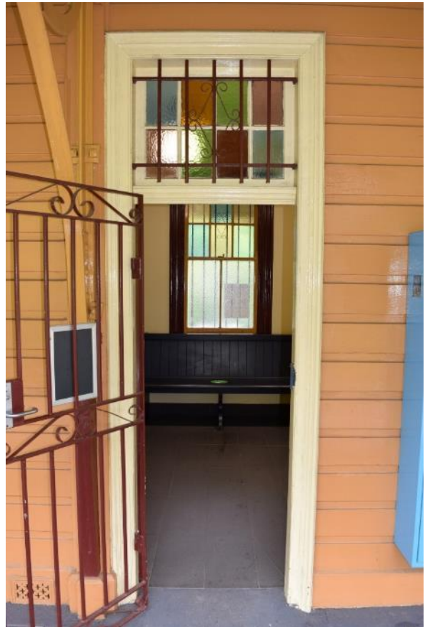
Figure 39 Closeup view of the station building door (Platform 2 waiting room)
