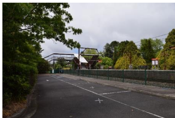
Figure 106 Overview of the informal kiss and ride area looking south
