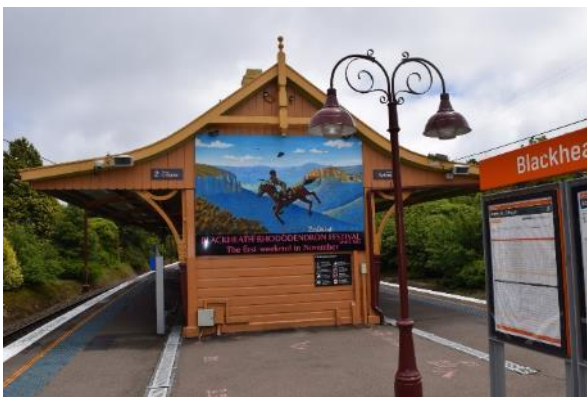
Figure 32 View of the south elevation of the main station building and mural
