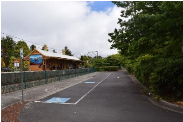
Figure 30 Overview of the main station building from the informal kiss and ride area
