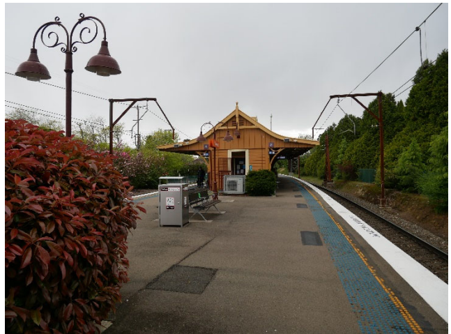
Figure 17 The Station building from the north (Source: Purcell, 15 October 2021).
