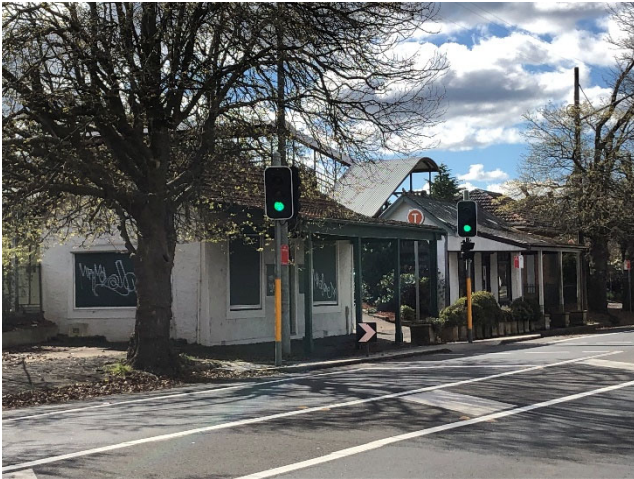
Figure 14 The pair of retail buildings on the Great Western Highway with the Station entrance between and footbridge beyond. (Source: Purcell, 22 September 2021)
