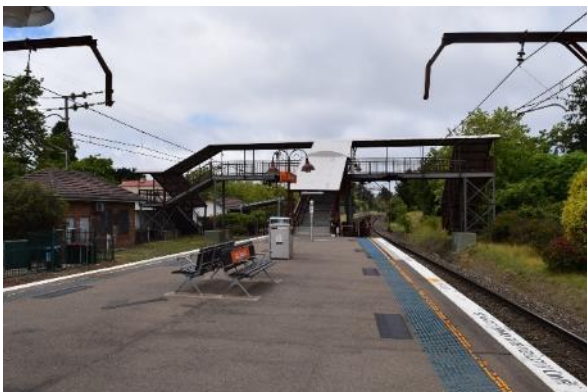
Figure 113 View of the platform and footbridge looking south
