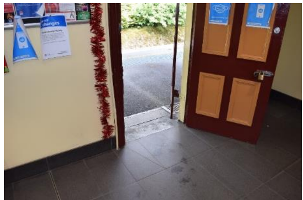
Figure 49 Closeup view of the west door and internal threshold
