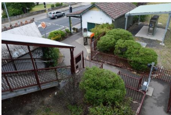
Figure 67 Overview of the level crossing
