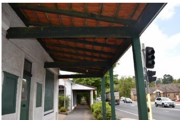
Figure 95 Closeup view of the south shop
