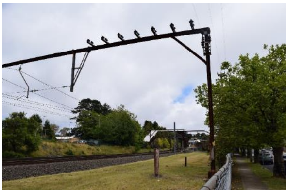
Figure 129 View of the precinct from the footpath and verge looking north
