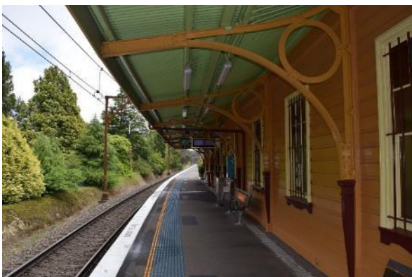
Figure 34 View of the west elevation looking north from the platform
