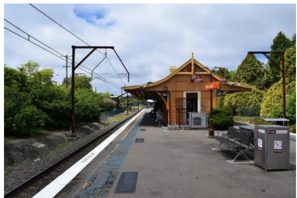
Figure 33 View of the north elevation of the main station building
