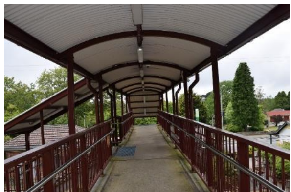
Figure 86 View of the footbridge deck looking east
