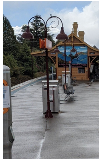
Figure 33 Existing light fitting. Note the interpretation of the detail to the top of the post. Purcell, 25 October 2021.
