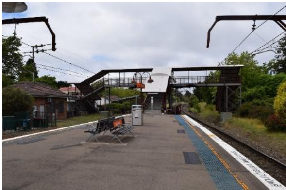
Figure 75 Overview of the footbridge
