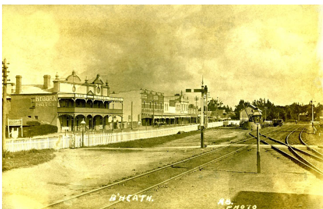
Figure 18 Retail buildings opposite the station on the Great Western Highway opposite the station. (Source: unknown, 'Blackheath Station', Australian Railway Historical Society (AHRS), 510025, supplied by client)
