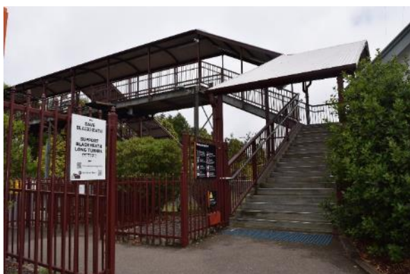
Figure 79 View of the east stairs
