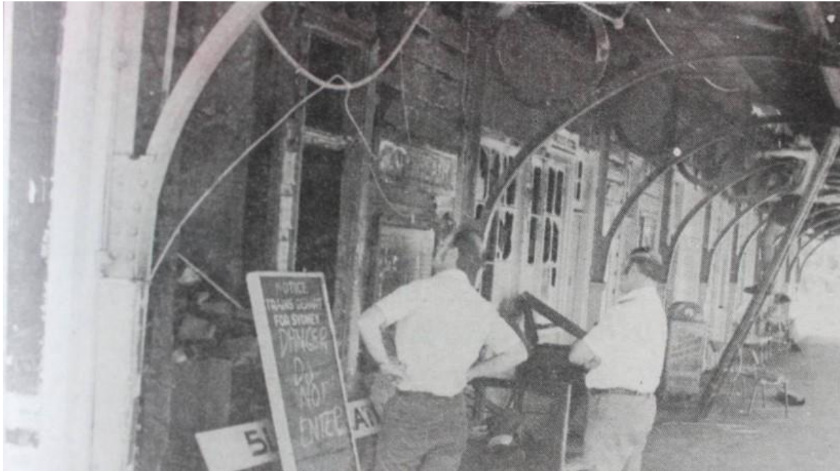
Figure 28 Photograph of the fire damage at Blackheath Station, 1985 Source: Lithgow Mercury, 2015
