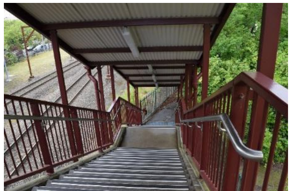
Figure 84 View of the west stairs from the footbridge
