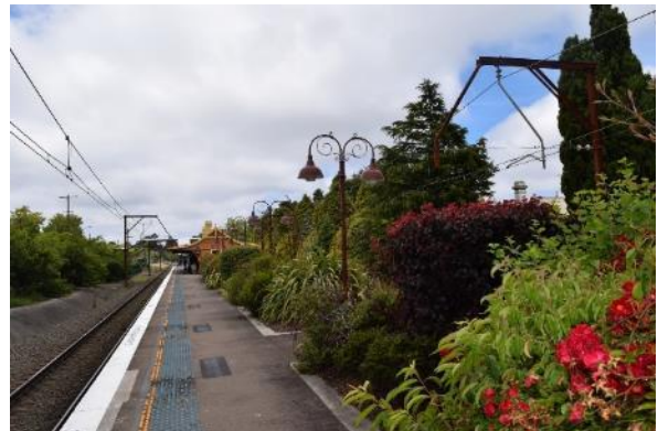
Figure 57 View of the platform looking south to the station building
