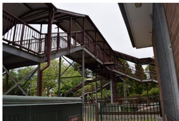
Figure 80 View of the footbridge
