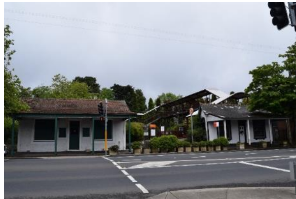
Figure 124 Overview of the shops and footbridge from Gardners Inn
