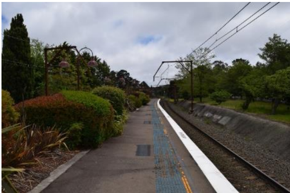
Figure 56 View of the platform looking north from the north end of the station building
