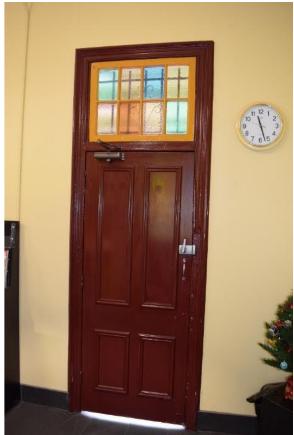
Figure 51 Internal overview of the east door at the General Waiting Room
