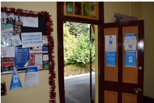
Figure 48 Closeup view of the west door and surrounding wall
