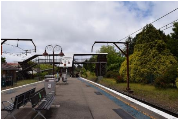
Figure 54 View of the platform looking south from the south end of the station building
