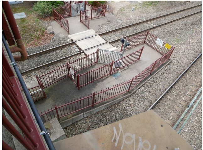
Figure 13 View from the footbridge to the level crossing (Source: Purcell, 15 October 2021).
