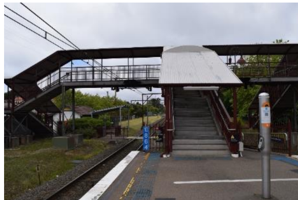
Figure 76 Overview of the footbridge
