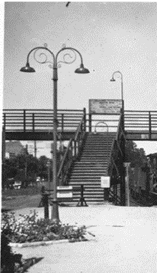
Figure 31 Detail of the light fitting in c.1950. (Source: unknown, 'Blackheath Station'; Australian Railway Historical Society (AHRs), 434363, supplied by client)
