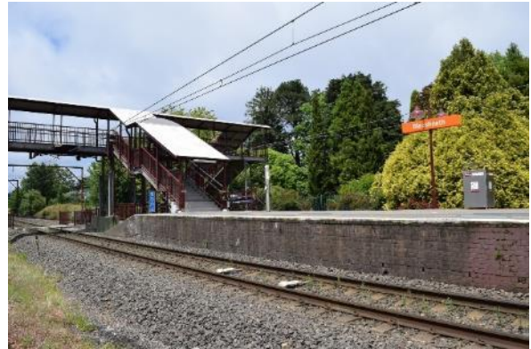
Figure 65 Closeup view of the brick platform edge
