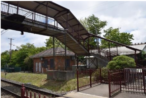
Figure 81 View of the footbridge from the level crossing
