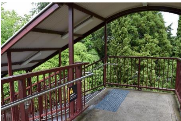
Figure 85 View of the west stairs from the footbridge
