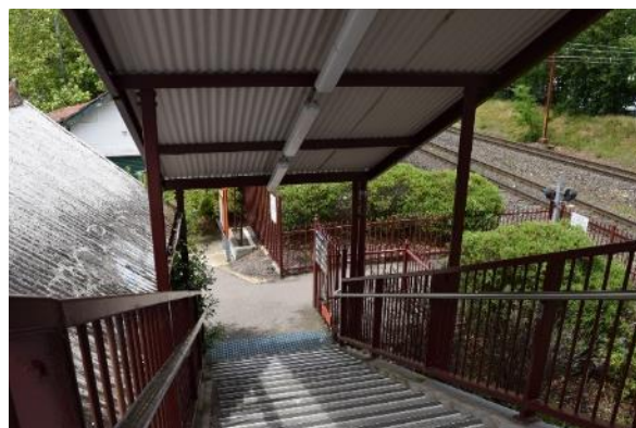
Figure 90 View of the east stairs from the footbridge
