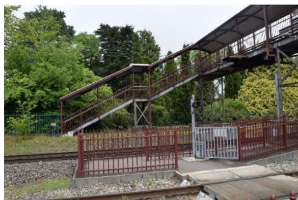
Figure 74 View of the level crossing
