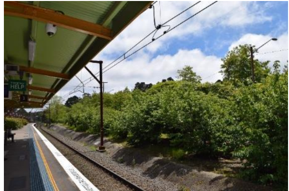
Figure 37 View of the east elevation awning looking north from the platform
