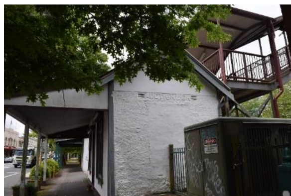
Figure 96 Closeup view of the north shop
