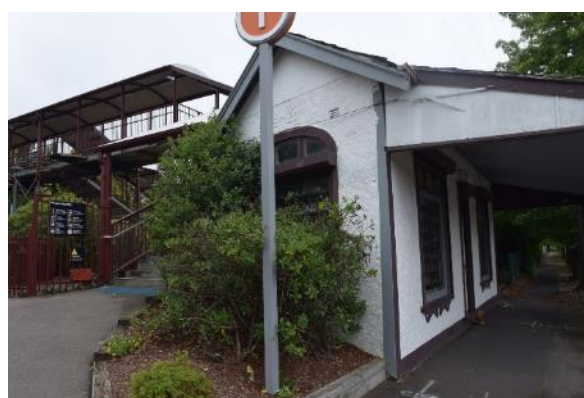
Figure 92 View of the north shop
