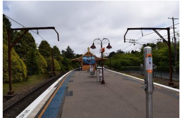
Figure 53 View of the platform looking north
