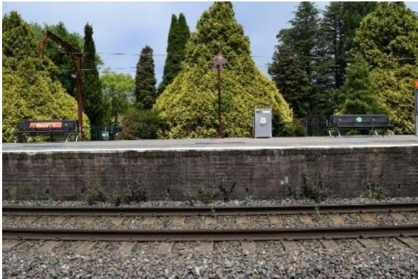
Figure 64 Closeup view of the brick platform edge
