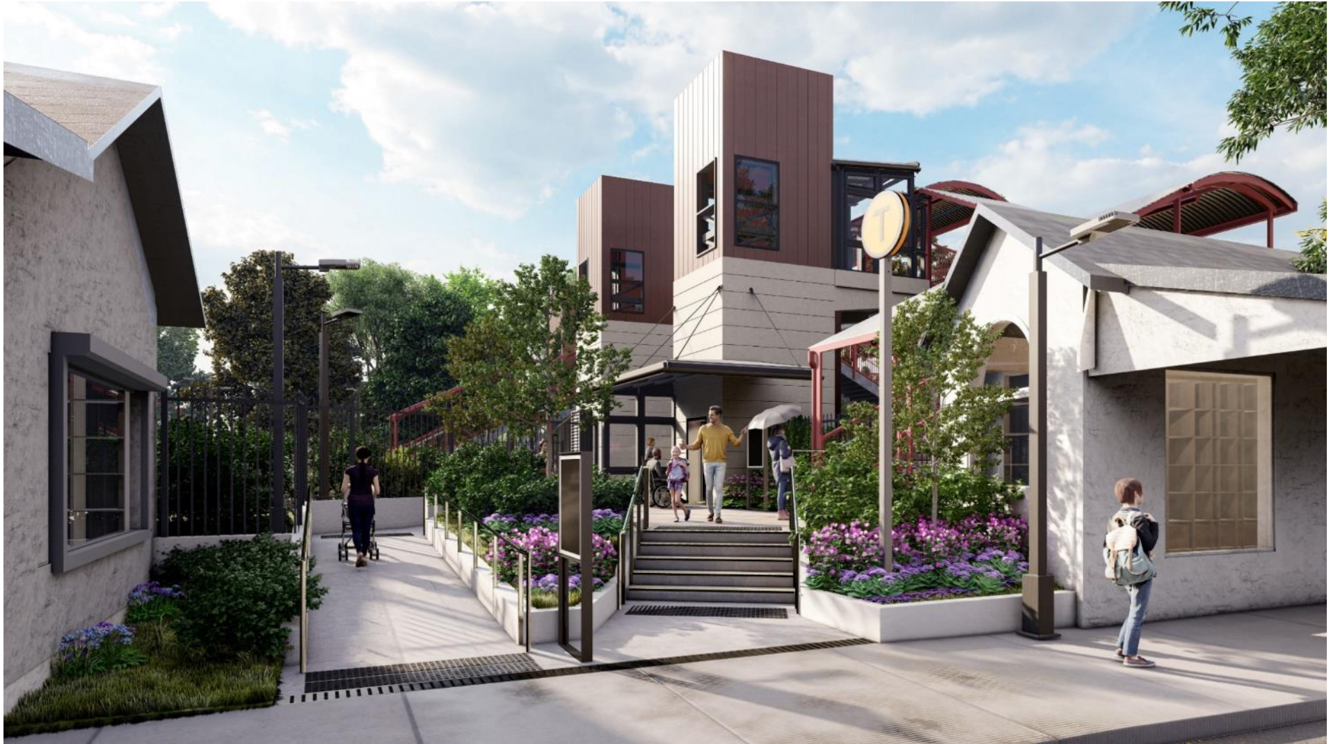
Figure 137 Architectural render of the Proposal. This is an artist impression and indicative only Source: Transport for NSW
