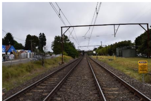
Figure 128 View of the railway line and precinct from the Bundarra Street level crossing
