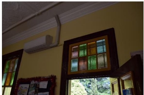
Figure 47 Closeup view of the door, wall and ceiling junctions
