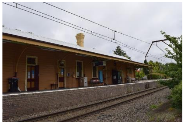
Figure 31 View of the east elevation of the main station building from the informal kiss and ride area
