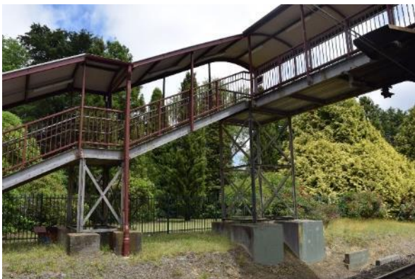
Figure 83 View of the footbridge from the level crossing
