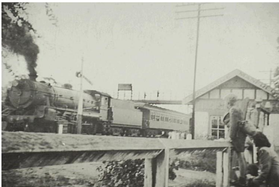
Figure 24 Photograph of Blackheath Station showing the overhead pedestrian bridge, 1947 Source: Blue Mountains Library, Resource ID 004082
