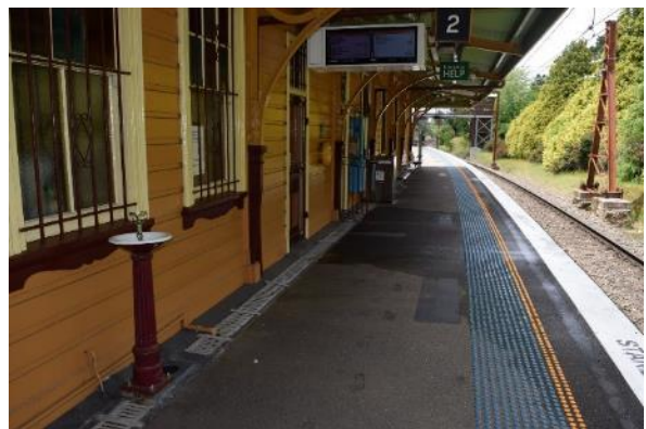
Figure 35 View of the west elevation looking south from the platform
