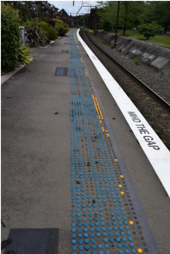
Figure 66 Closeup view of the platform surface, tactile ground surface indicators (TGSIs) and platform edge
