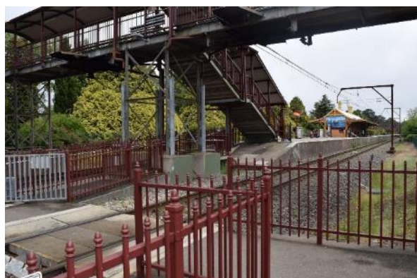
Figure 73 View of the level crossing
