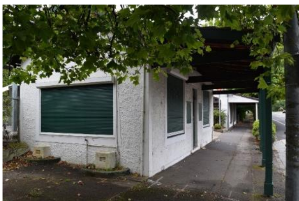
Figure 93 View of the south shop
