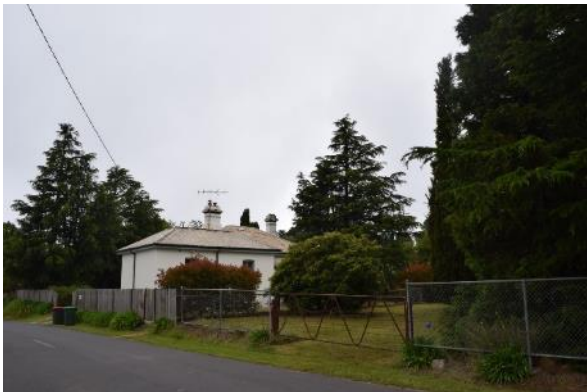
Figure 117 View of the Former Station Master's House from Station Street
