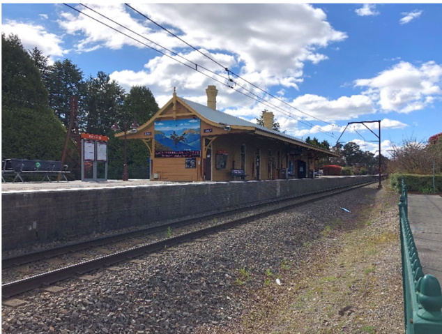
Figure 16 The Station building and island platform from the Great Western Highway Carpark looking north. (Source: Purcell, 22 September 2021)
