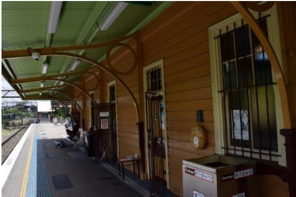
Figure 36 View of the east elevation looking south from the platform
