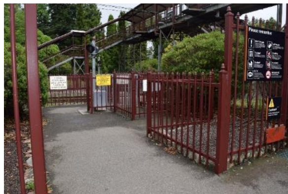
Figure 70 View of the level crossing from the main entrance
