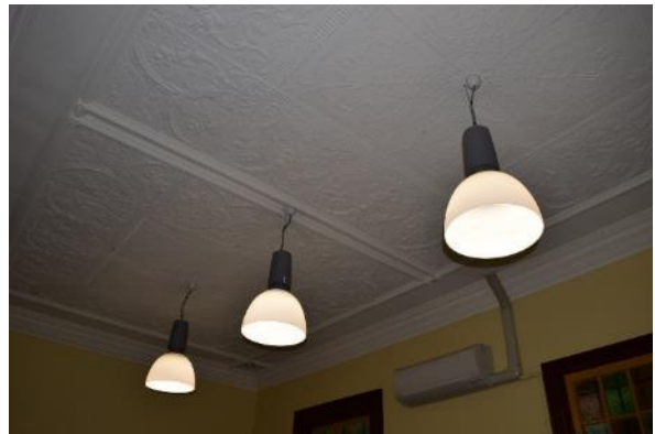
Figure 45 Overview of the pressed metal ceiling and light fixtures
