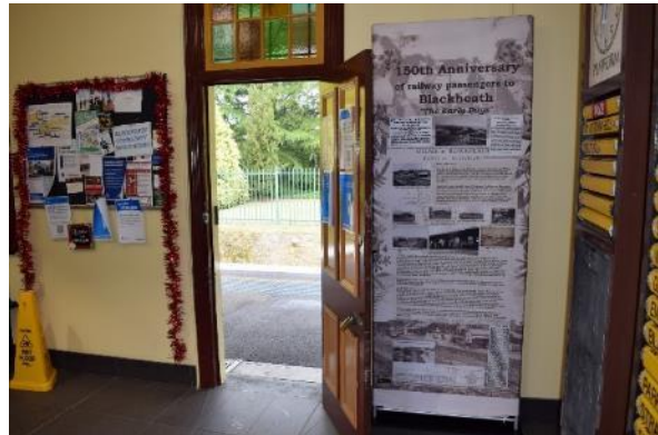
Figure 41 View of the internal west wall and door
