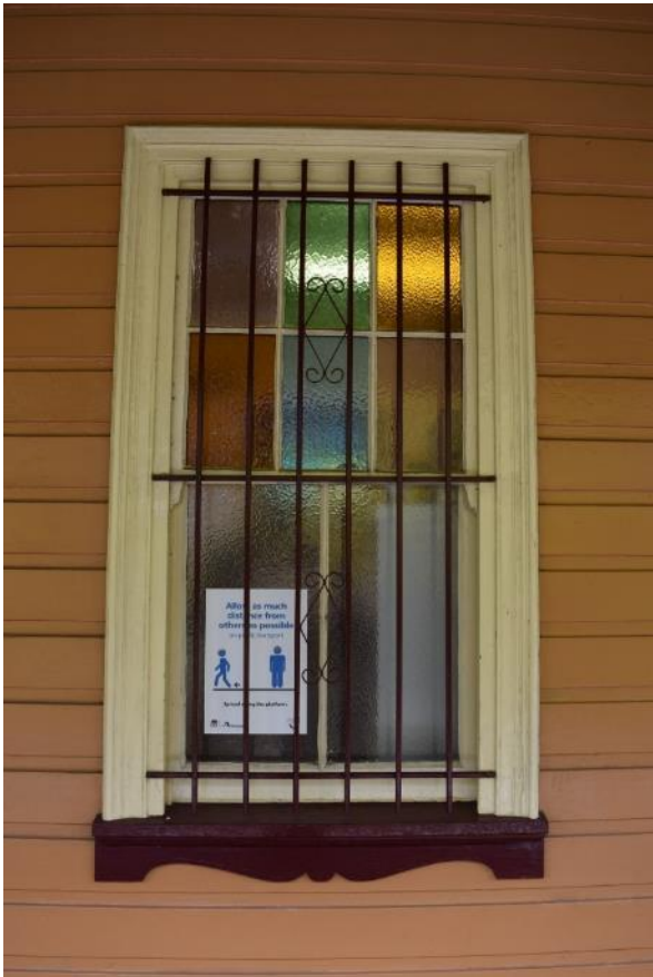
Figure 38 Closeup view of the Platform 1 waiting room window.
