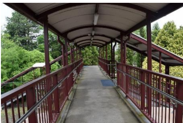
Figure 87 View of the footbridge deck looking west
