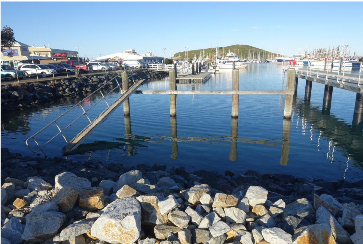
Figure 2-8 Existing timber structures on site. The timber piles and walers are proposed to be retained. The timber catwalk is proposed to be removed.
