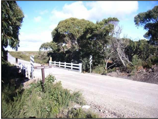
Sundown Creek bridge (Segment B).
