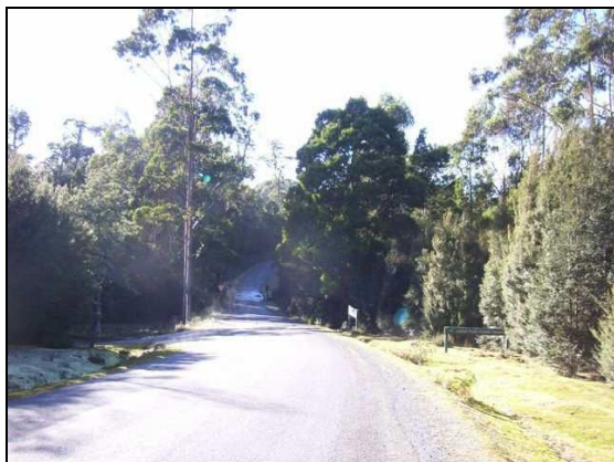
The existing sealed section through the Julius River Forest Reserve
