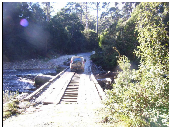
Rapid River bridge (Segment K)
