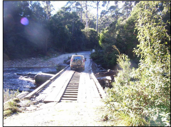
Rapid River bridge (Segment K)
