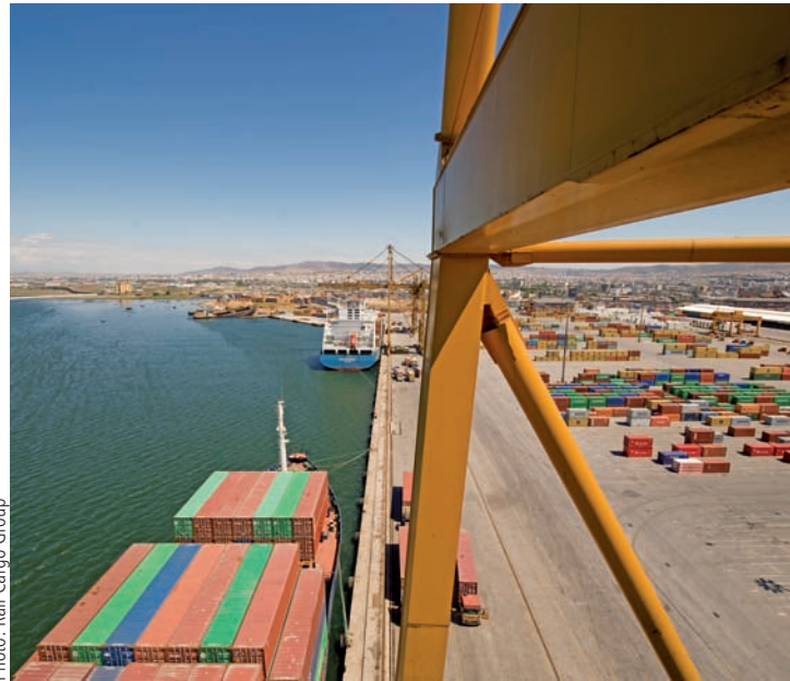
Photo: Rail Cargo Group
