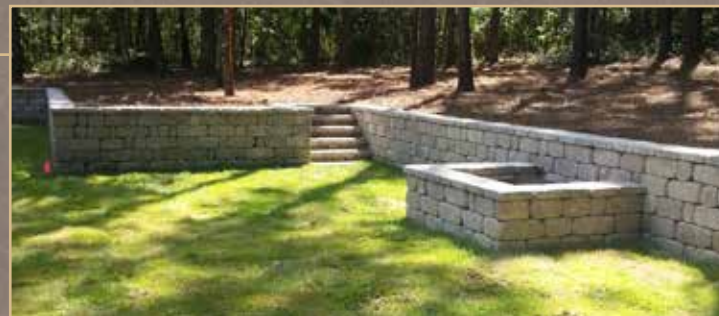
GRAVITY WALL Near Vertical Detail
