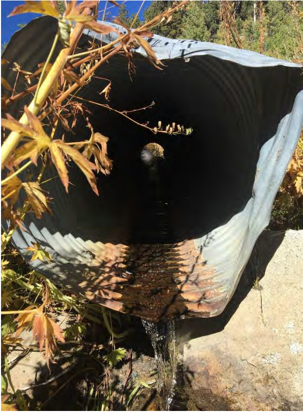
On Mountain Culverts 9-25-18:
