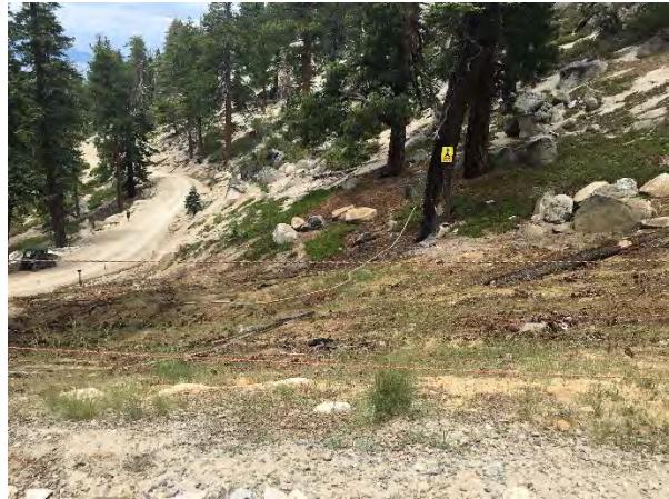
Hand Grenade Chute 2018: erosion resistance significantly improved with revegetation
