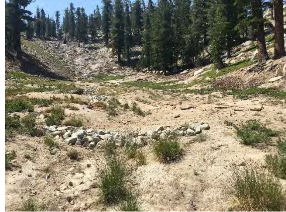
Ridge Bowl After: gully regraded with riprap protection of outlets
