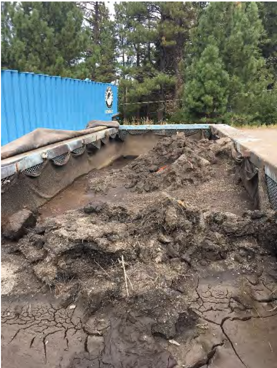
CA Base Storm Drain Annual Maintenance with Clean Harbors August 2018:
