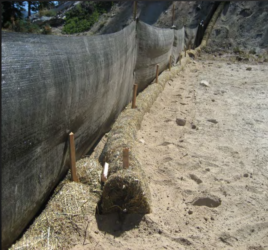
Straw wattle with silt fence
