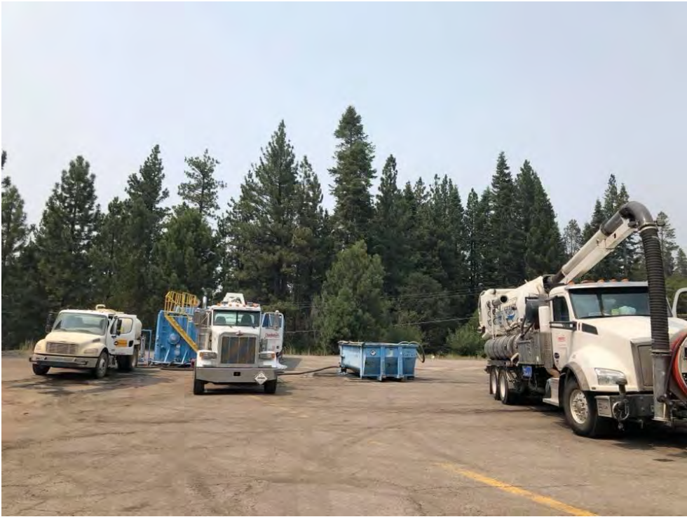
CA Base Storm Drain Maintenance with Clean Harbors August 2018:
