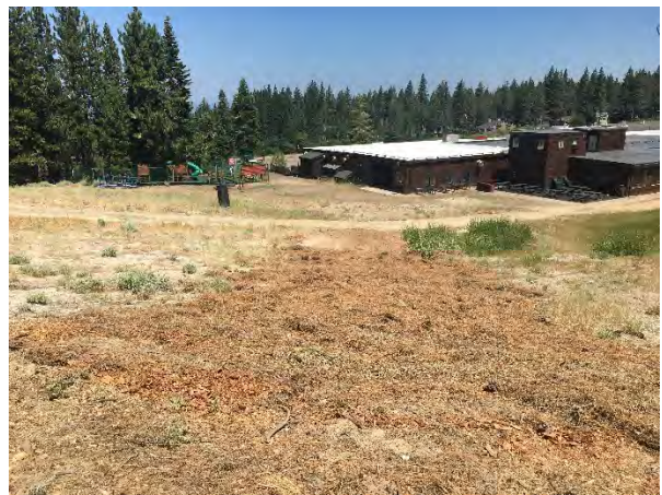
After: Area tilled and mulched to provide erosion resistance and effective cover.
