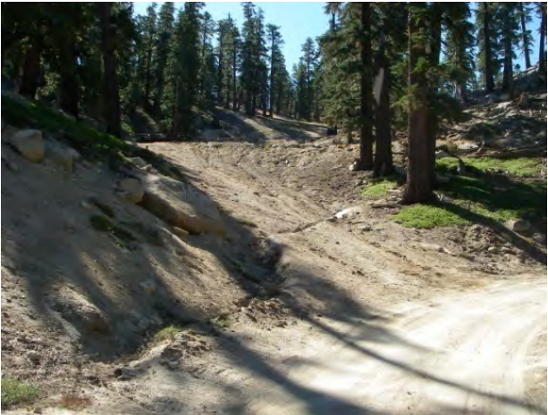
Hand Grenade Chute 2017 Before: bare soils, rilling, water bar minimally functioning
