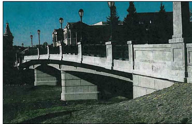
EXAMPLE OF DECORATIVE PEDESTALS AND LARGE BLOCK RUNNING BOND FORM LINER PATTERN ON COLUMNS AND WINGWALLS
