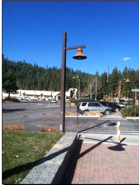
EXISTING ROCK WALLS AND STREET LIGHT STANDARD AT TAHOE CITY VISITORS CENTER
