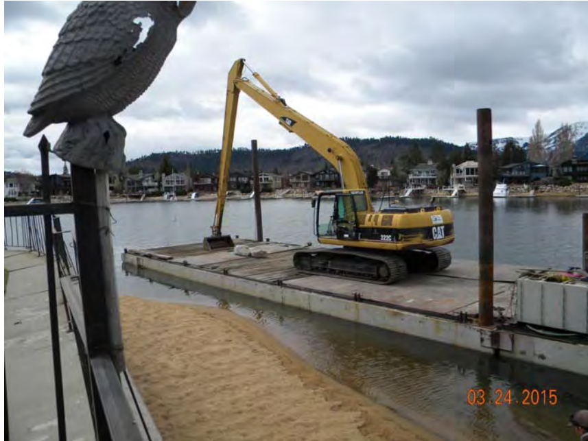
Mechanical dredging equipment at Tahoe Keys ( https://www.tkpoa.com/images/photos/projects/dredging/dredging5348.JPG )
