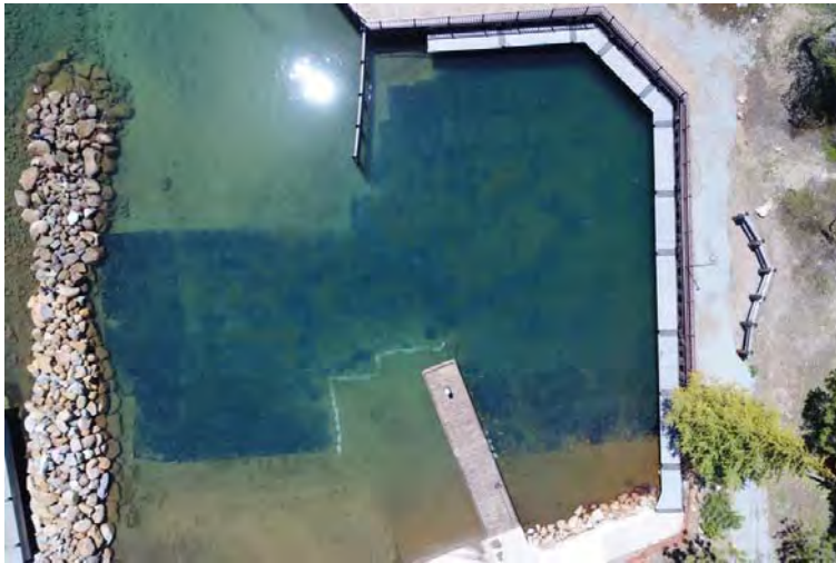
Benthic barrier array in the Tahoe Vista boat launch
