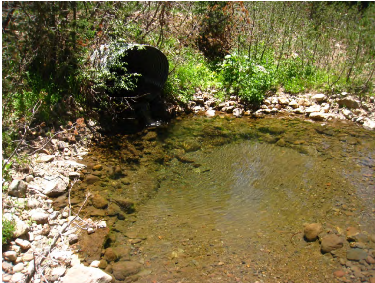
GPS WP#416 Hanging culvert on stream crossing, Webber Lake Road 120°26'10.582"W 39°26'49.093"N
