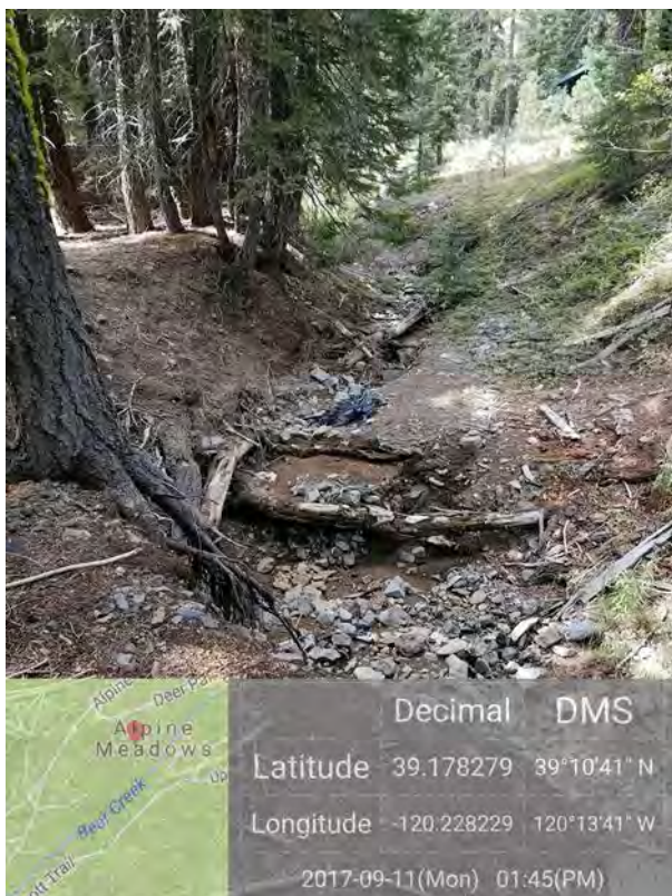
Eroded tributary channel below Alpine Meadows Road
