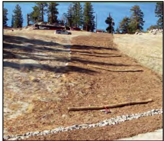
Restoration treatment following installation of a water line (IERS, 2009)
