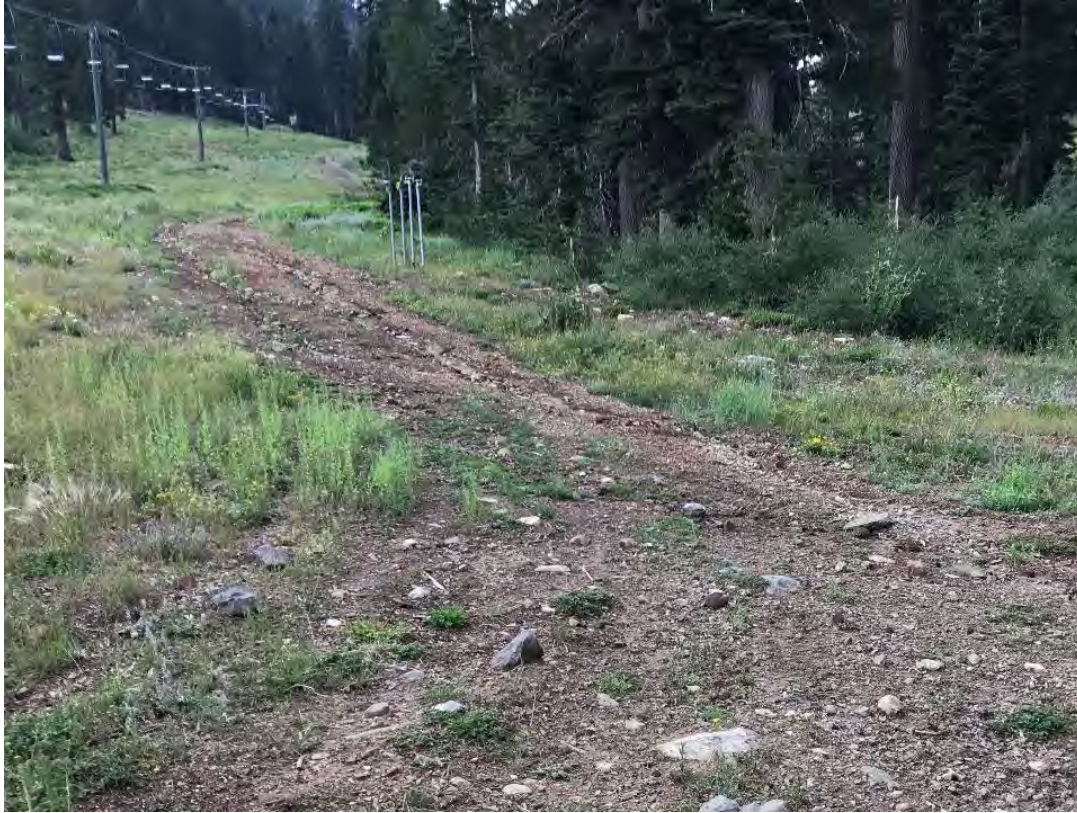
Figure 4-24 Erosion along water lines, adjacent to Meadow Chair, Alpine Meadows Ski Area, Tahoe National Forest, Placer County, California.
