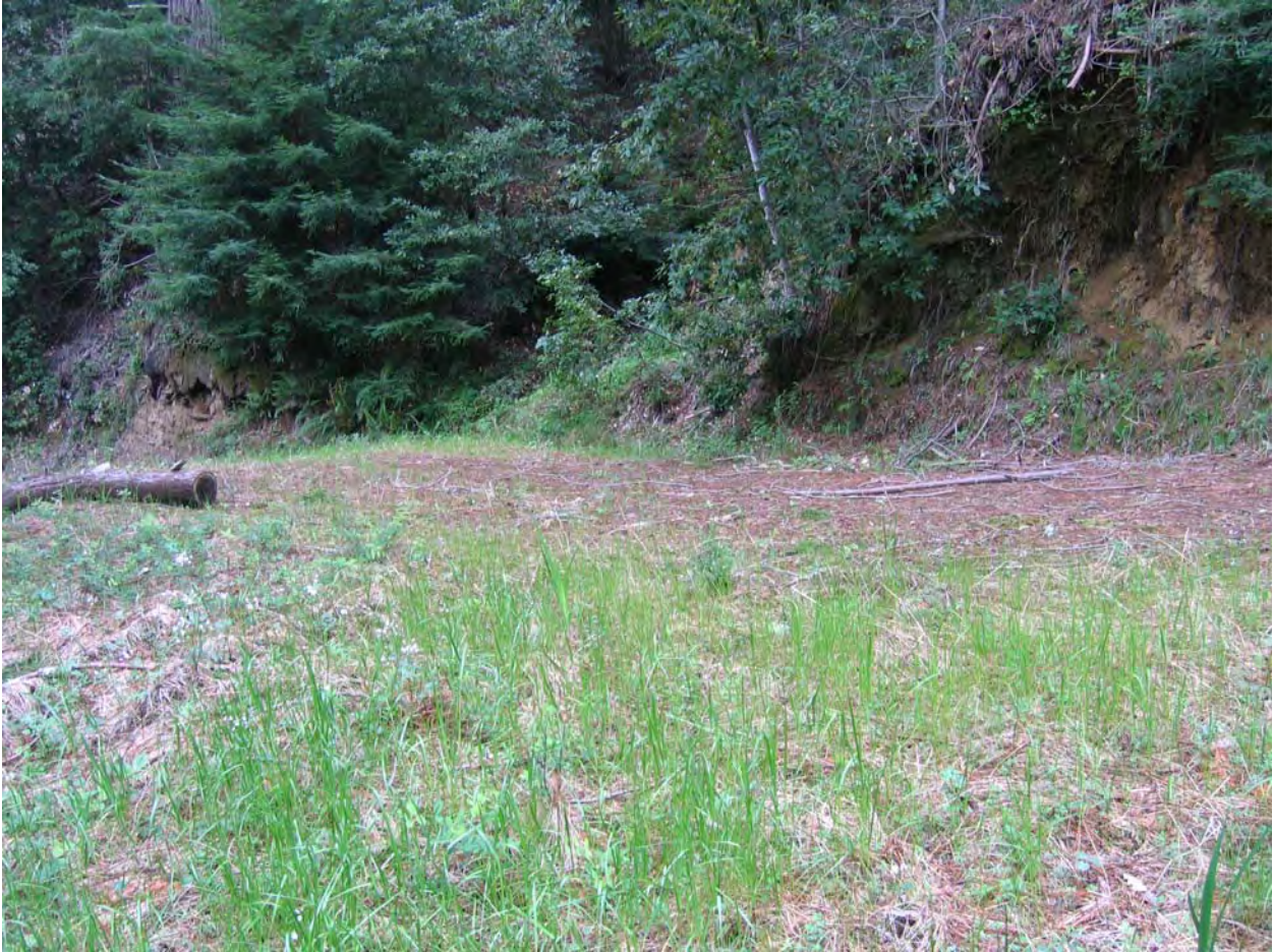
Photo # 9: A properly built rolling dip.
