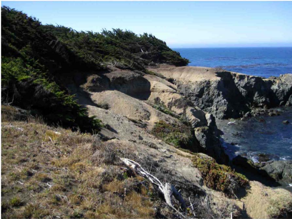
Figure 4. Eroding layer of unconsolidated sediments between the Monterey cypress and the coastal bluff in Unit # 17.
