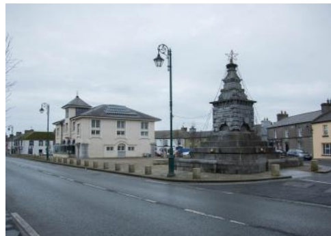
fig. 11.1 Abbeyleix crescent town square and market house
