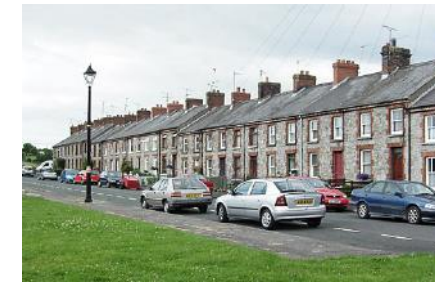
fig. 17.5 (above) Mill Housing, Bessbrook
