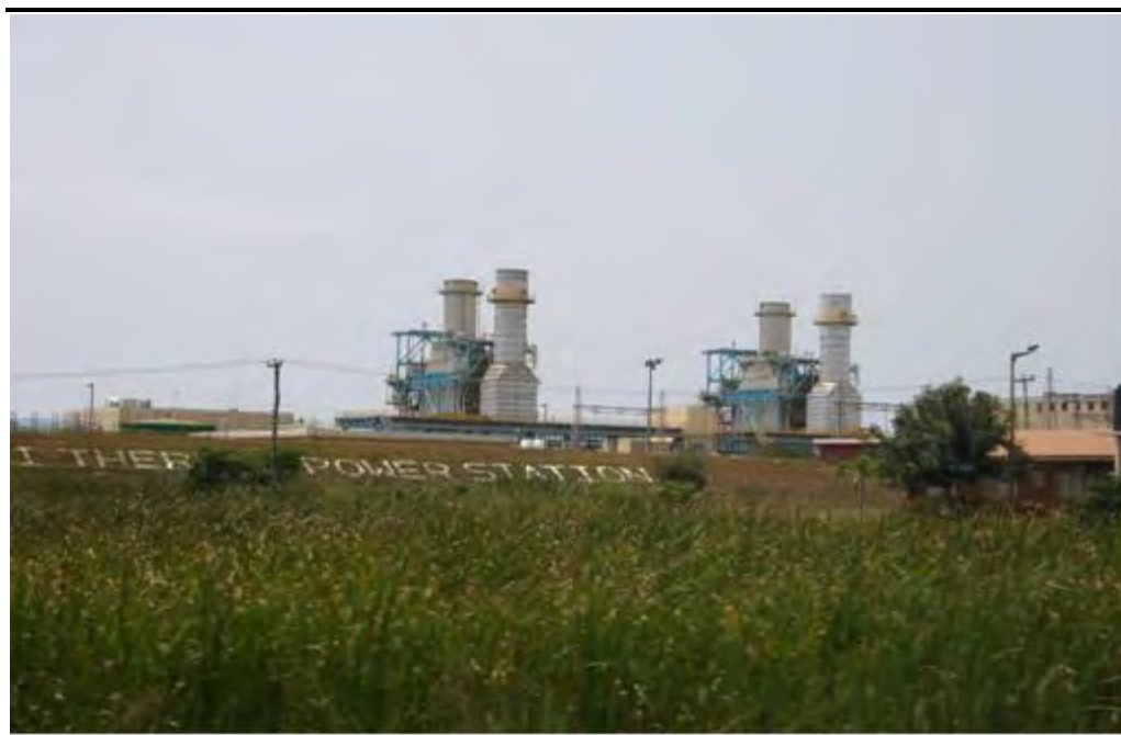
Figure 6.13 Takoradi Thermal Power Plant
