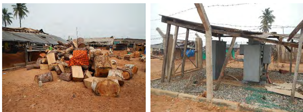
Figure 6.15 Firewood and Electricity Transformer
