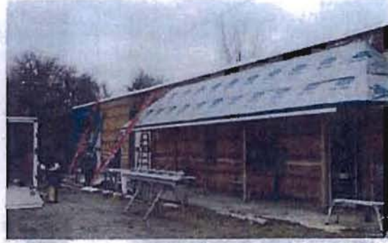
Prepping for the new siding, on the new facility.
