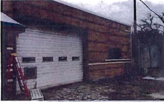
Removing the old siding, from the new facility.
