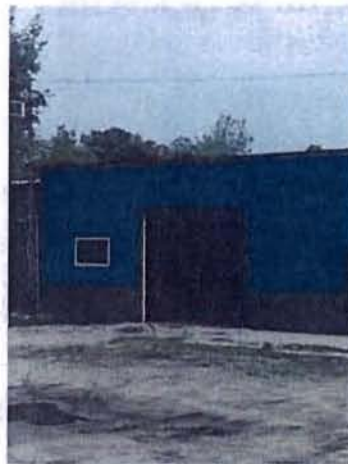
New siding, on the new facility.
