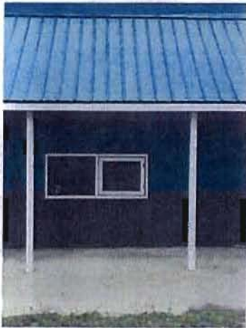
New siding, on the new facility.
