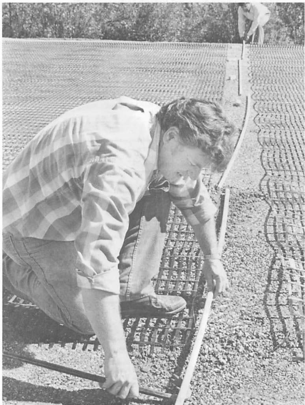
Dr. Tom Kinney, associate professor of civil engineering, works on a project studying the feasibility of using geotextiles to prevent permafrost problems in Alaska highways. UAF photo/Sam Winch
