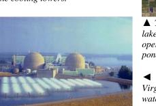
The Grand Gulf Nuclear Station in Mississippi uses a natural draft cooling tower normal during operation and mechanical type cooling towers (upper left) in event of an accident.  $\nabla$
