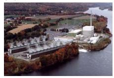
The UHS can be the same nearby lake, river, or ocean used by the nuclear plant to absorb waste heat during normal operation or it can be a different, dedicated water source. However configured, the UHS is supposed to provide all of the nuclear power reactor's cooling water and makeup water needs for the first 30 days of an accident.
