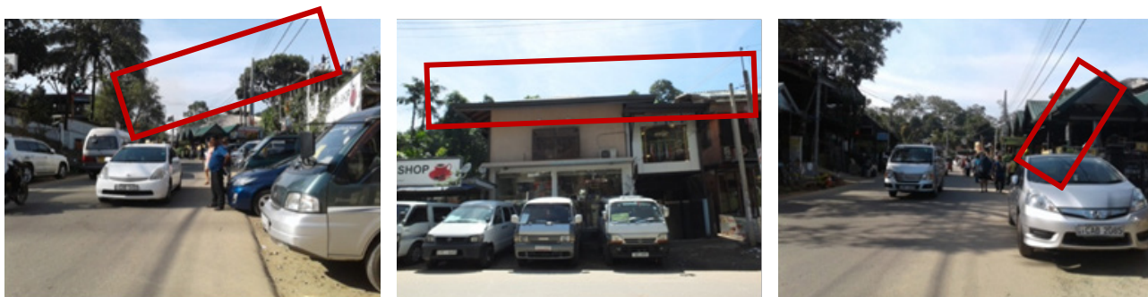
Figure No 5.12 : Irregular Car parks and the electricity cables that mar the appearance
