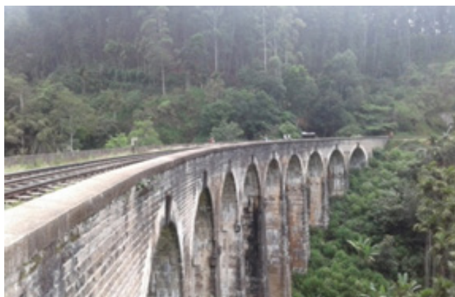
Arch - Bridge in Demodara
