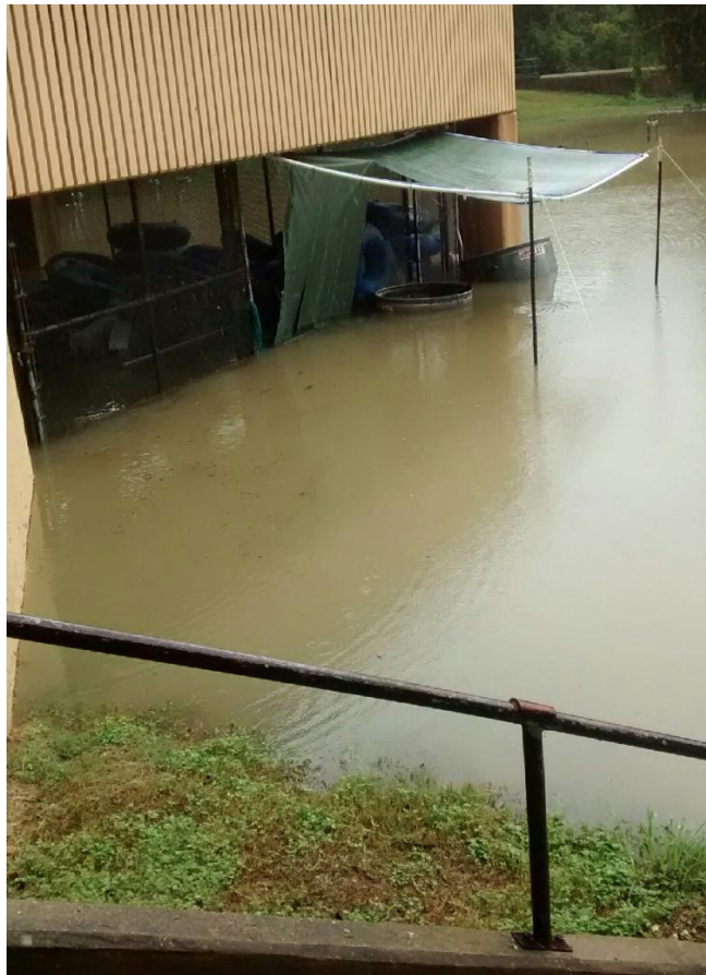
Figure 11. Photo showing flood levels in the stream channel area at Texas State University in San Marcos on September 26, 2016. All stream channels were flooded about 3ft above their normal water level.
