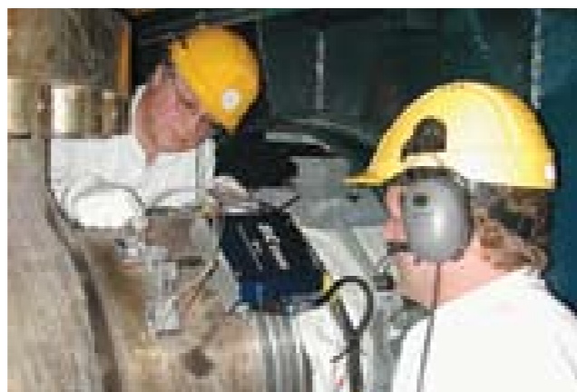
Control of work quality, procedures established in advance, and developed internal inspections are key elements of the safety culture.
