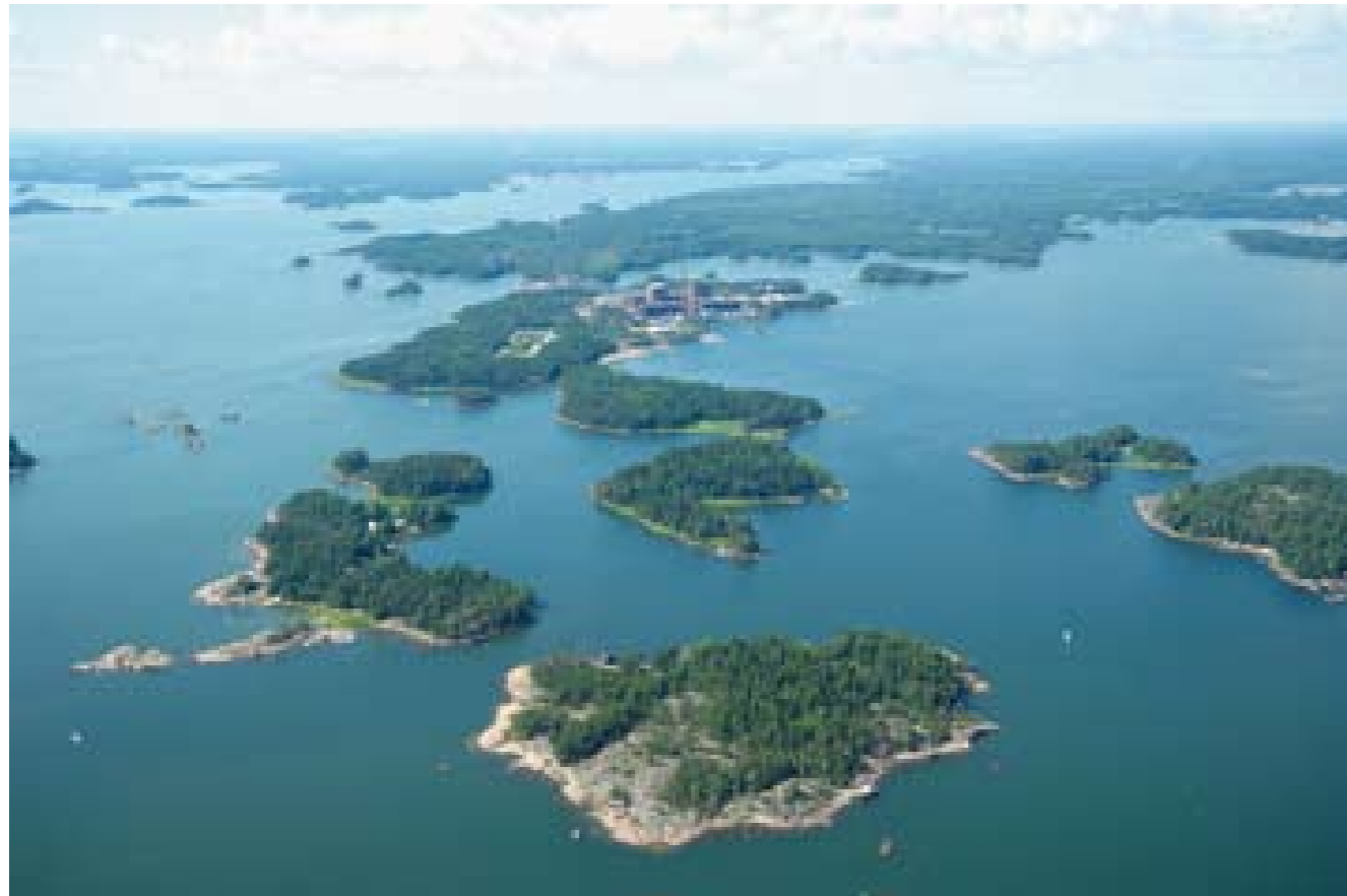
Figure 7-7. An aerial photo of the Loviisa Power Plant with its surroundings taken from southeast. In front Myssholmen, on the left side of the power plant Hudöfjärden and on the right Hästholmsfjärden.
