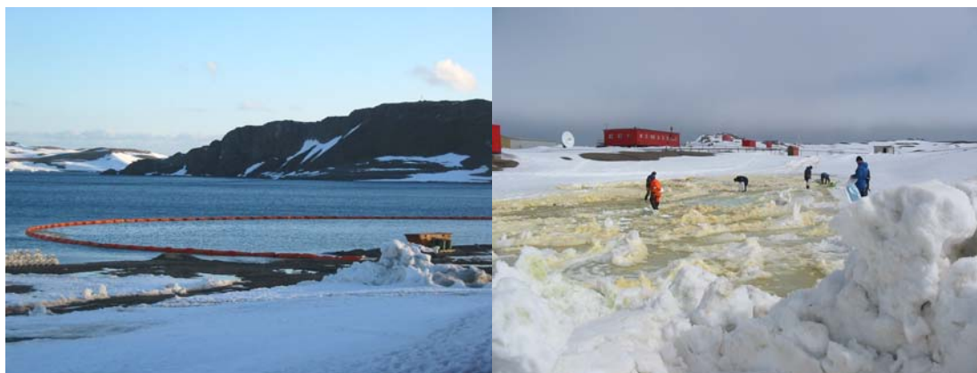
Fig. 4.2.-16a & b: Measures taken after a severe oil spill (a) oil boom at Maxwell Bay (b) removal of the oil impregnated snow by members of the station (photos: Bellingshausen)
