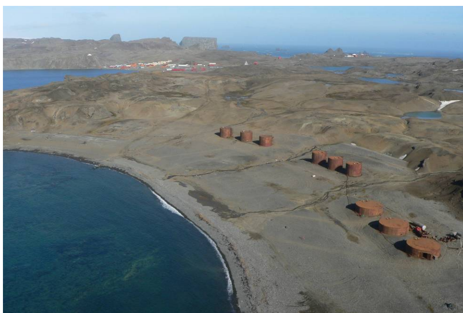
Fig. 4.2.-13: Neftebasa – large oil tank farm (photo: Buesser)
