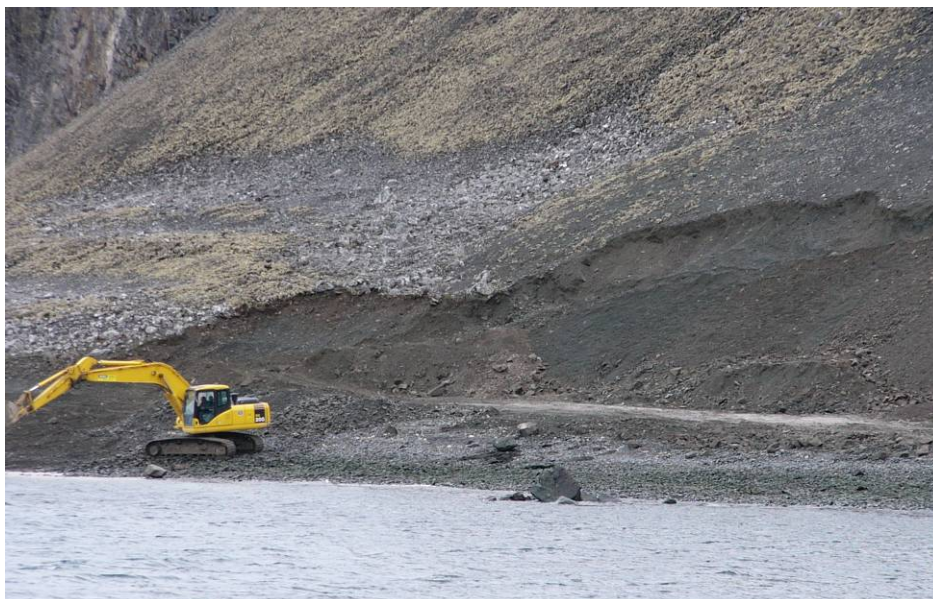
Fig. 4.2.-69: Quarry No. 3 with lichen growing on the storm petrel breeding ground (photo: Peter)
