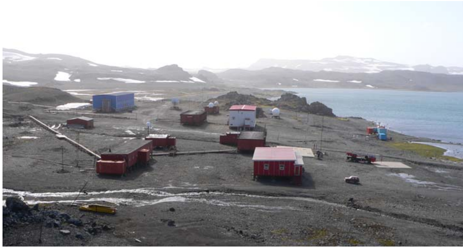
Fig. 4.1.-2: Chinese station Great Wall in the southern Fildes Peninsula (photo: Buesser)
