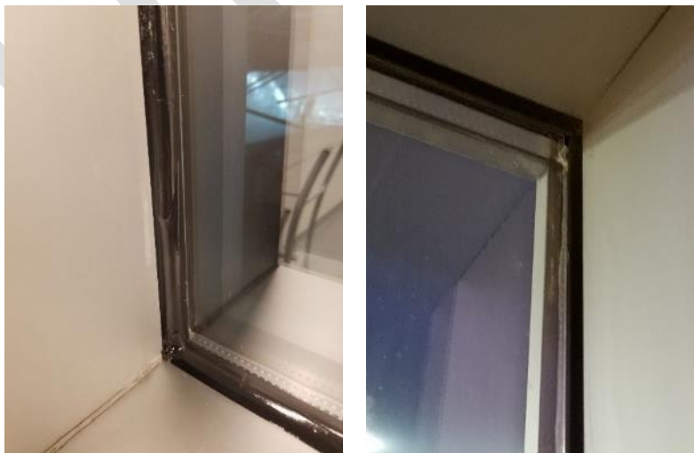
Figure 12: Installation of SRF in attached methods.
