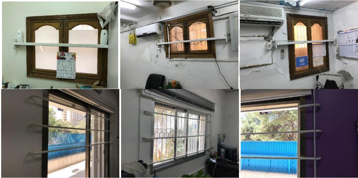
Figure 14: Examples of rigid catcher system, anchored horizontally.
