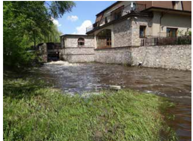
Figure 1. Renovated water mill before transformation into SHP
