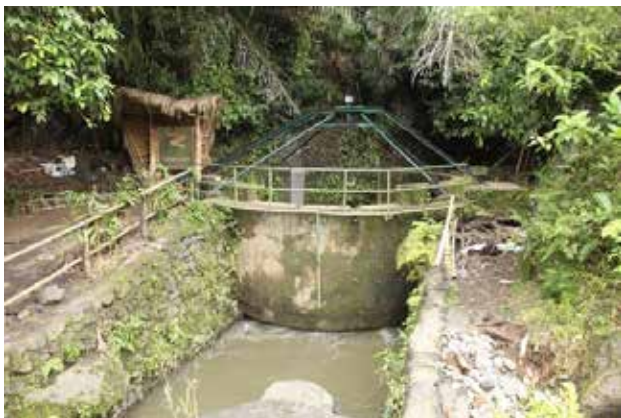
Figure 3. Civil works of the 13 kW turbine in Green School Bali, Indonesia
