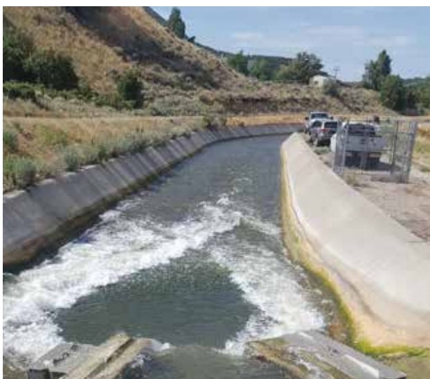
Figure 4. Smart Free Stream in an irrigation canal, USA
