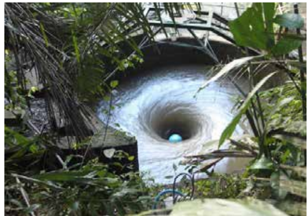
Figure 6. Installation and commissioning of the Green School turbine
