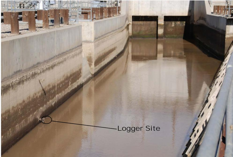
Photo 16 – Fish Screen Bay Temperature Monitoring Site
