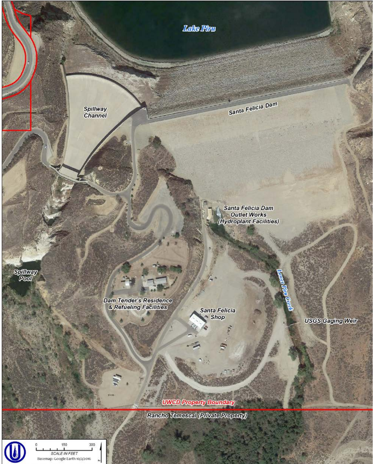
Figure 2-2 Santa Felicia Dam and Spillway
