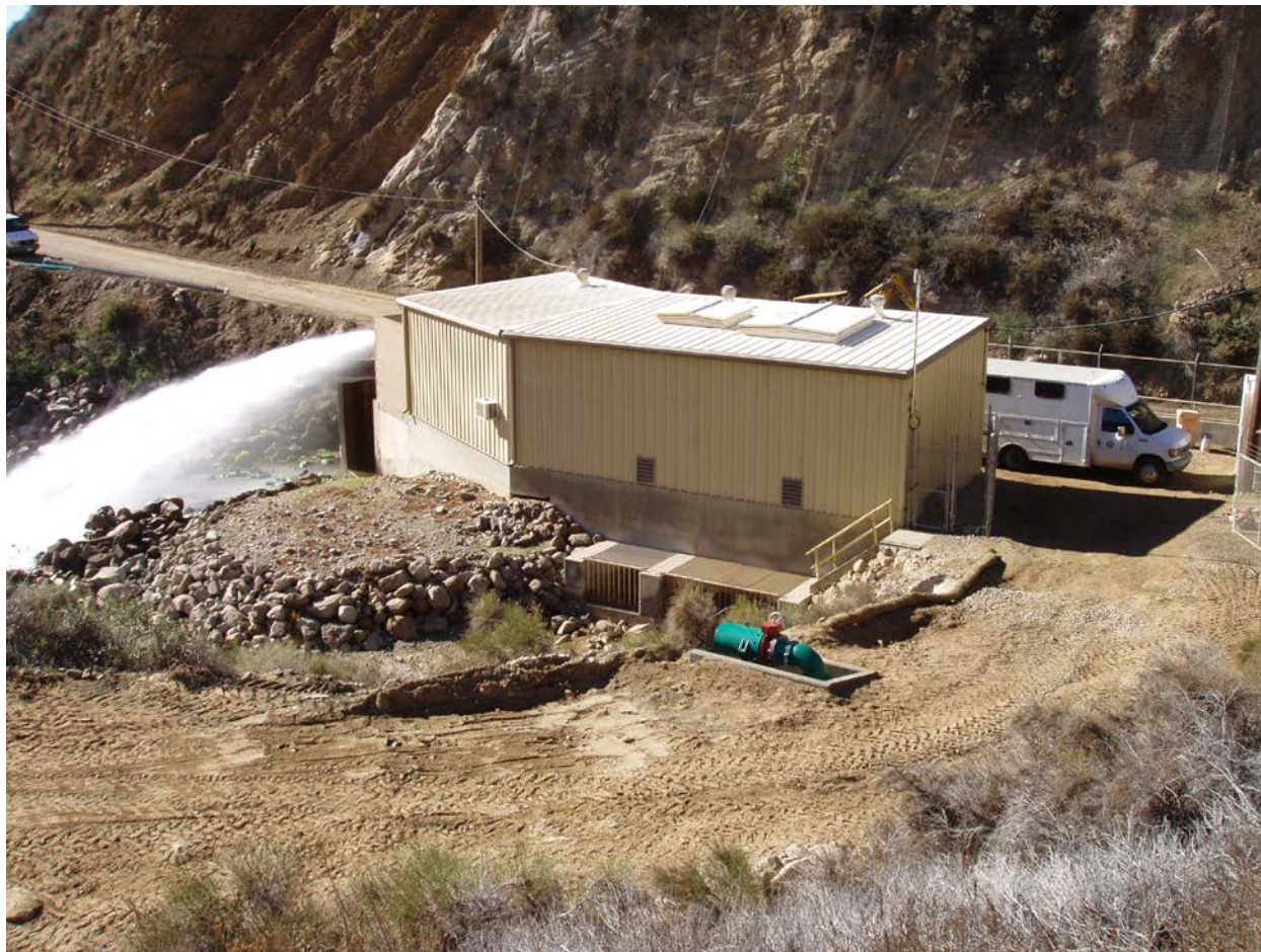
Figure 2-11 Low-Flow Release through the 12-Inch West Valve (the East Valve is shown in the foreground)
