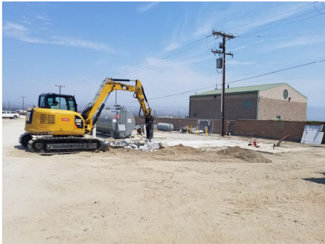
Demolition of Existing Generator Pad
