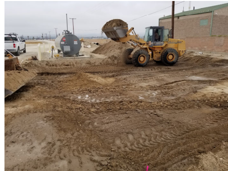
Over-Excavation and Compaction for the new Pad
