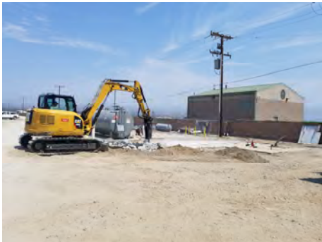
Demolition of Existing Generator Pad
