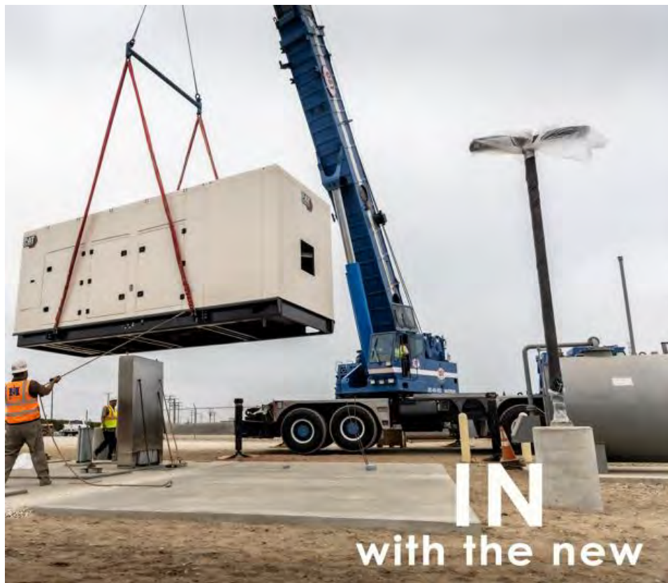
Figure 10 OH System Backup Generator Project – New Generator Installation
