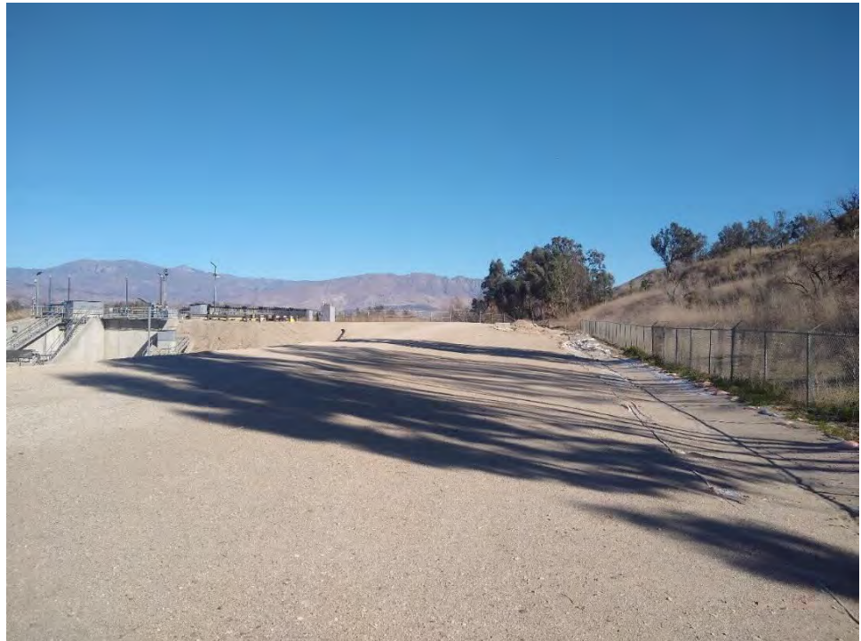
Photo 2: Facing northeast from the northern portion of Upland Work Area 2 (January 14, 2021).
