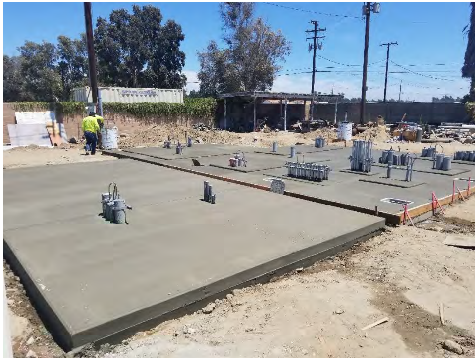
Figure 8 OH System Backup Generator Project – Concrete Pad Placement
