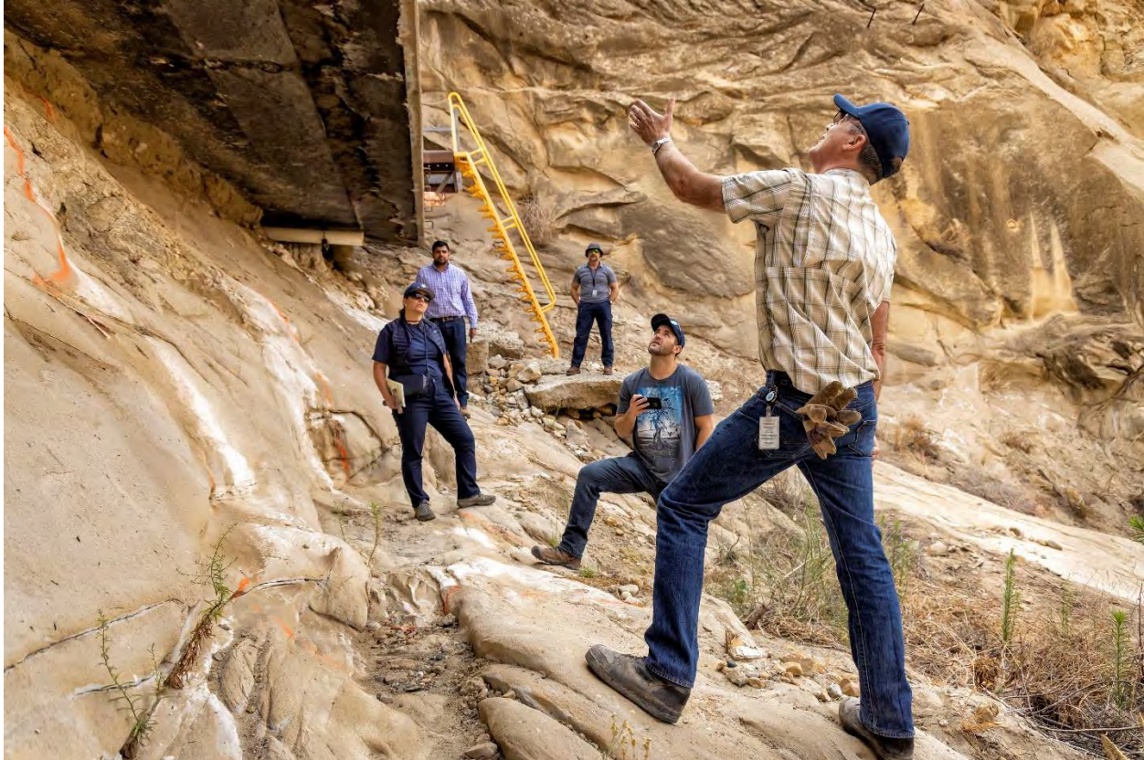
Figure 3 DSOD Inspection of the Spillway Discharge Channel on August 16
