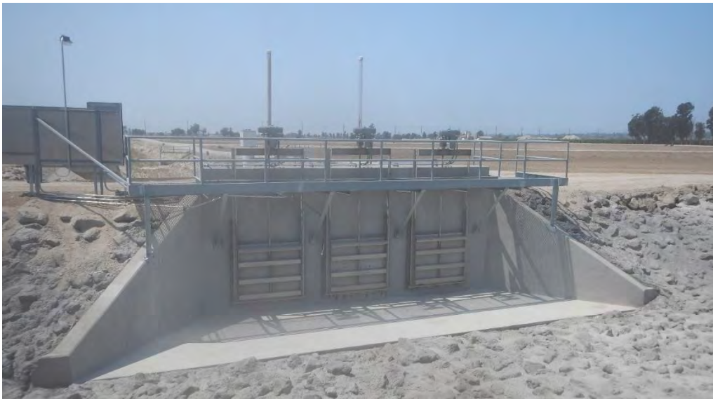
Figure 6 Grand Canal Headworks – Construction Complete
