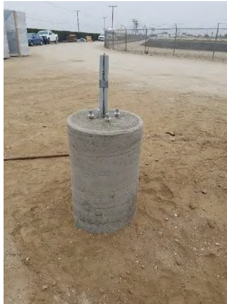
Figure 9 OH System Backup Generator Project – Light Pole Foundation Replacement
