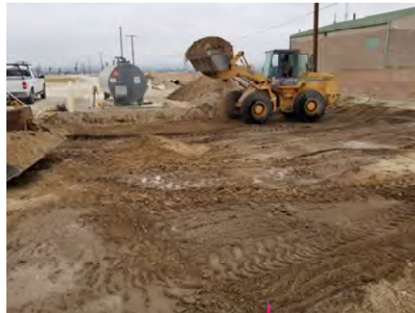
Over-Excavation and Compaction for the new Pad
