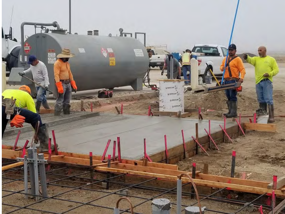
Figure 7 OH System Backup Generator Project – Concrete Pad Placement
