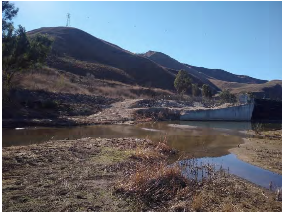
Photo 4: Facing southwest from the Upstream Work Area (January 14, 2021).
