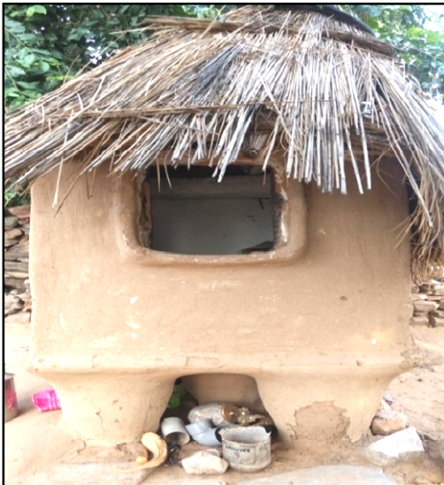
Food storage hut ( Obra )
