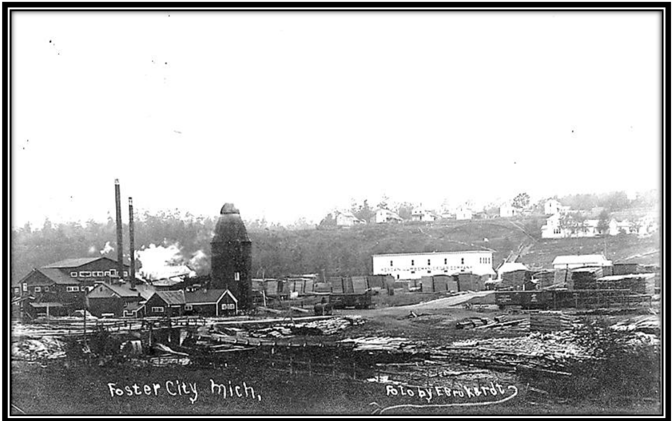
Morgan Lumber & Cedar Company Sawmill, Foster City, Dickinson County, Michigan, ca. 1910-1915: This unused real photo postcard view identified as “Foster City, Mich.” probably dates between 1910 and 1915 and shows the Morgan Lumber & Cedar Company sawmill at the left with the sawdust burner, the Morgan Lumber & Cedar Company store near the center and a portion of Boarding House Hill in the background in the right. Note the bridge across the Sturgeon River in the left foreground in front of the sawmill. This view was taken by E. Brukardt (Ernest Robert Brukardt, amateur photographer who worked as a railroad station agent in Felch). [William J. Cummings]
