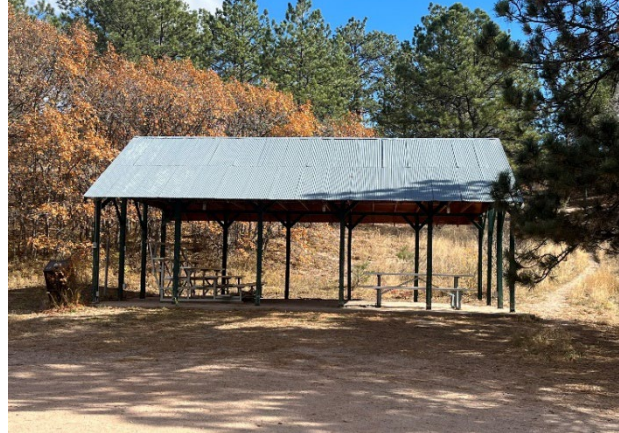
Figure 7: Photo of the Pavilion adjacent to Kettle Lake #3 (October 24, 2022)
