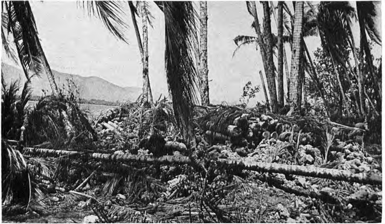
LOG AND CORAL BUNKERS opposed the American advance. More than 70 of these well-camouflaged works formed strong points on the main enemy defense line between Kia Village and Munda Airfield. Until artillery and naval gunfire cleared the thick growth, the bunkers were difficult to locate.
