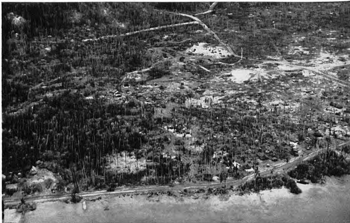
BETWEEN LAMBETI PLANTATION AND MUNDA POINT lay flat ground which, less than a month after the fall of the airstrip, became a desolate camp site. From the "quarries" near the center of this picture came the coral with which Seabees and engineers paved roads and landing strip. (Navy Photo.)
