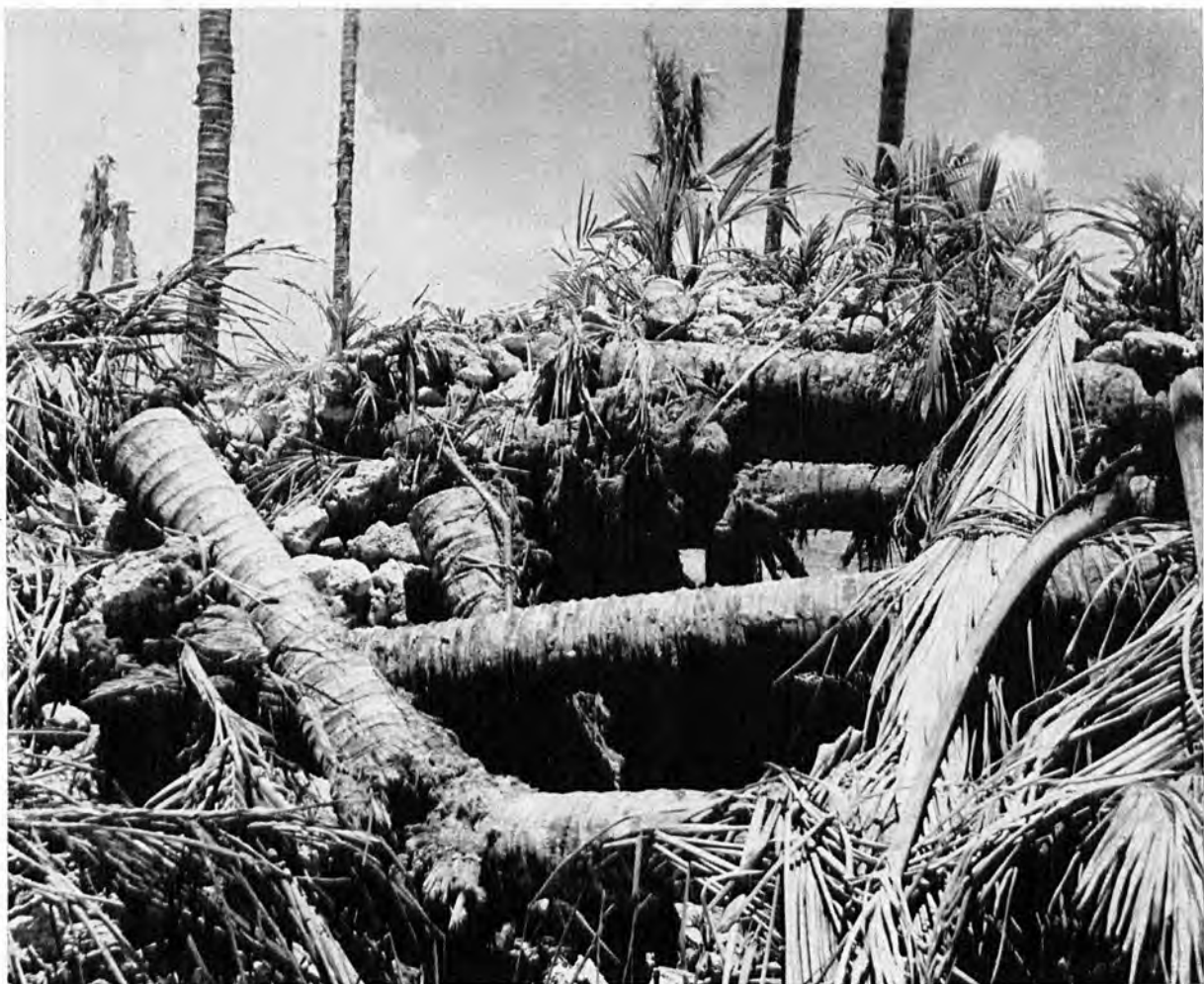
LOG AND CORAL BUNKERS studded the coast of Kolombangara. After the Japanese withdrawal from the island in early October, Marine artillerymen landed to study the effects of their fires. This particular bunker had received a direct hit from a 155mm shell.
