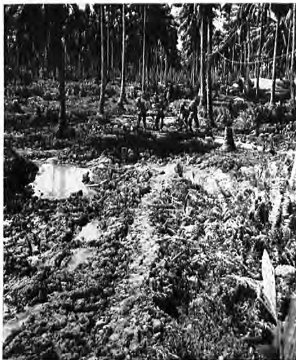
RAIN AND HEAVY TRAFFIC TURNED ROADS INTO QUAGMIRES but indefatigable Seabees worked tirelessly and soon had stalled vehicles moving again. Here a group corduroys a road that appears to be an impassable mud hole.
