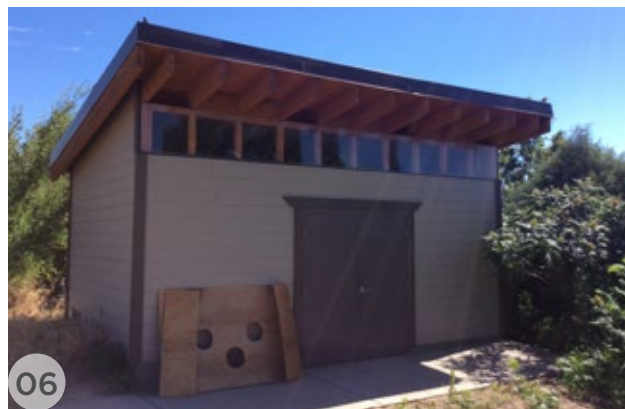
06 Storage shed near the Utah House
