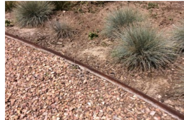
Gravel path with steel edging
