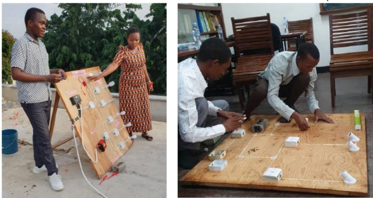
Figure 4. Attendees of the PV training during PV systems installation exercise 2022. (IPPS TAN:01/2)
