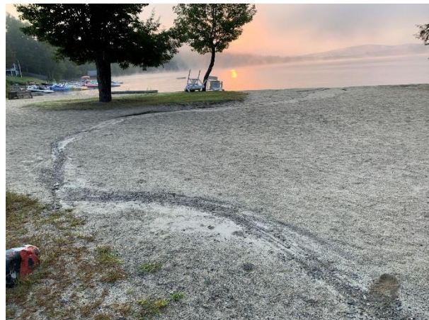
Photo 16. Dewey Beach erosion from uncontrolled road drainage Sep 2022. Credit: Barbara Chalmers.
