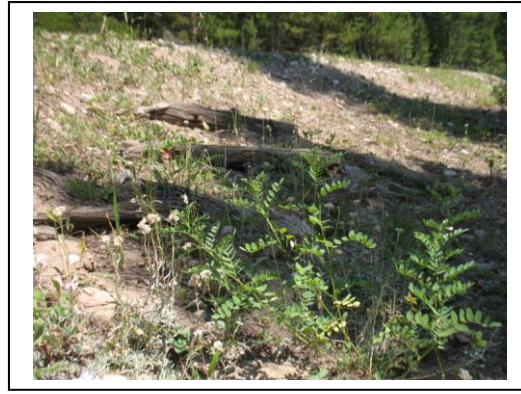
Figure 15. Sandy or gravel loams and sparse recolonization are evident at most roadcut sites. By M. Kirkpatrick.
