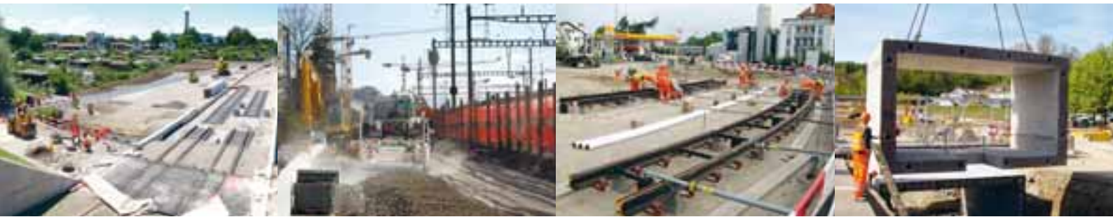
Rail track construction adjacent to family garden area
