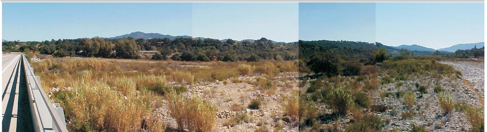
Figure 5.5-4: Panoramic view of Highway 150 Bridge Slurry Disposal Site Sub-site 2
