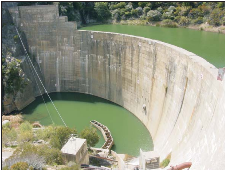
12. View of the dam, fish ladder, reservoir, and beginning of the Ventura River (Reach 6).
