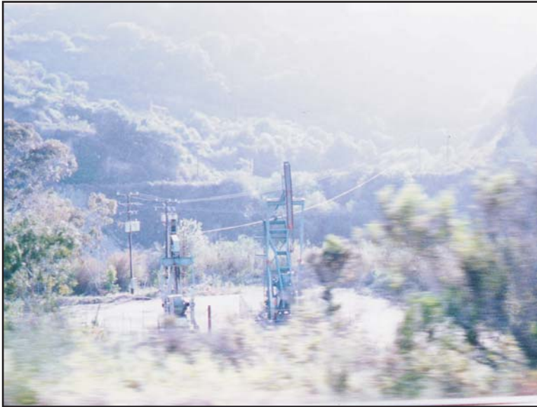
4. From SR 33 facing west view of the oil fields and tanks located in the northern portion of Reach 2b.
