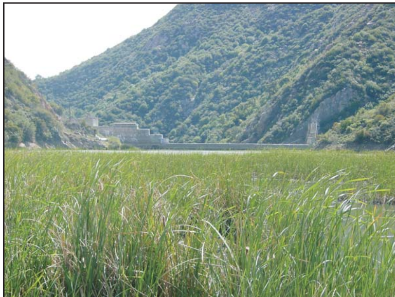
15. Close up of the top of the dam and surrounding slopes and vegetation (Reach 7a).
