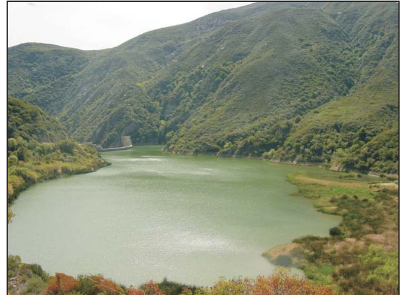
14. View of the top of the dam and reservoir area from Matilija Road (Reach 7a).
