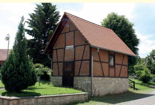
Brunnenhaus in Burkersroda
