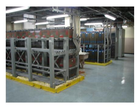
Figure 2. The -48V VLA battery strings are approximately 190 KWh each.
