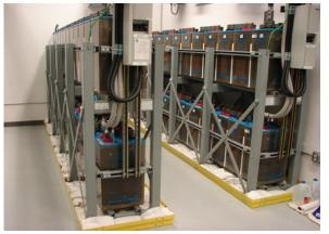
Figure 5. Planned exemptions for lead-acid batteries to be closer than 3 feet from walls or other obstructions would make the installations above permissible. Separation criteria for other technologies must be followed.
