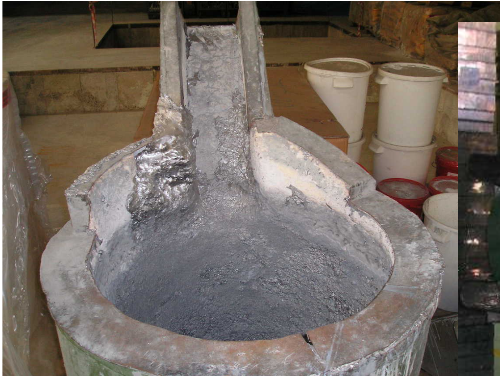
Refractory ladle: Before
