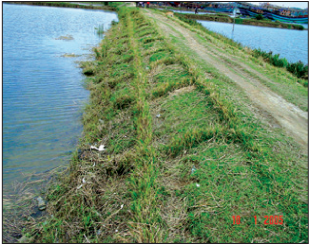
Photo 24a: Vetiver, installed in a cross-hatched pattern, protects shrimp pond dikes in Quang Ngai.
