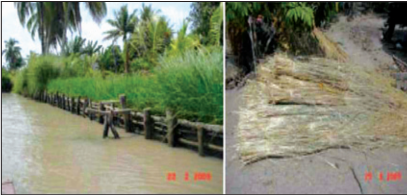
Photo 31: Left: Vetiver reinforces a wooden structure along a river; right: cut vetiver leaves make string for use as rice binding.
