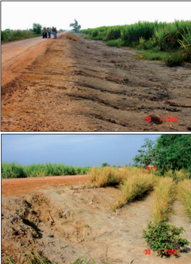
Photo 21: Before (upper) and after (lower) vetiver installation in extreme acid sulfate soil on an embankment in Tien Giang province, Vietnam.
