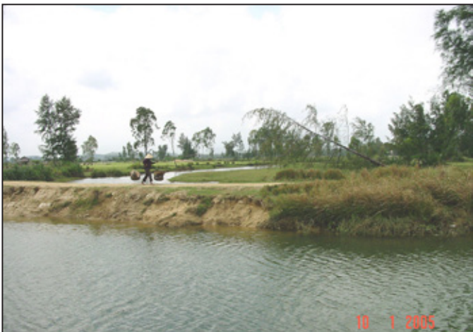
Photo 25: The right section of this rural road in Quang Ngai is protected by vetiver; the left section is unprotected.
