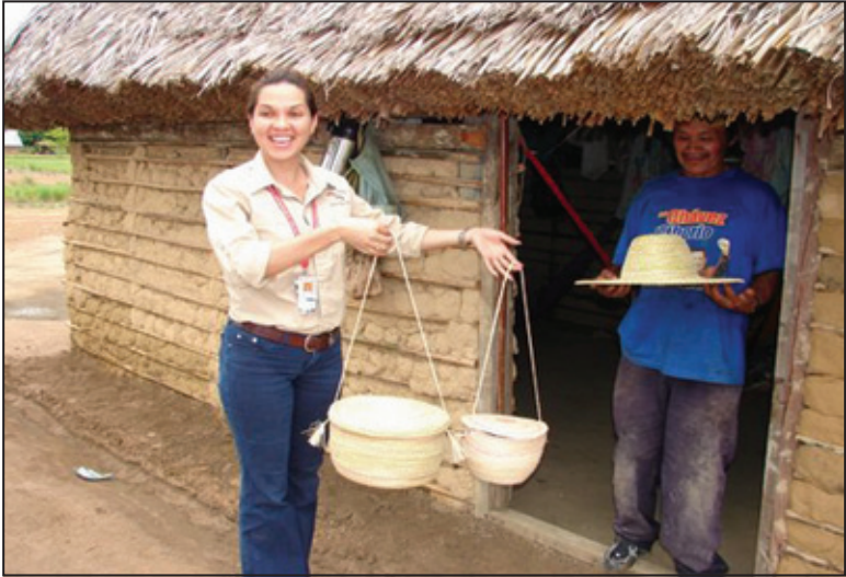
Photo 30: Roof thatching in Venezuela.
