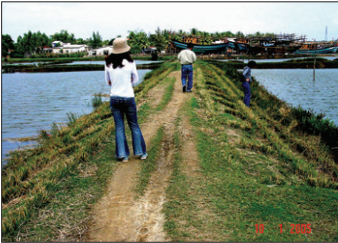
Photo 24b: Vetiver, installed in a cross-hatched pattern, protects shrimp pond dikes in Quang Ngai; photo shows both left and right side of dike.
