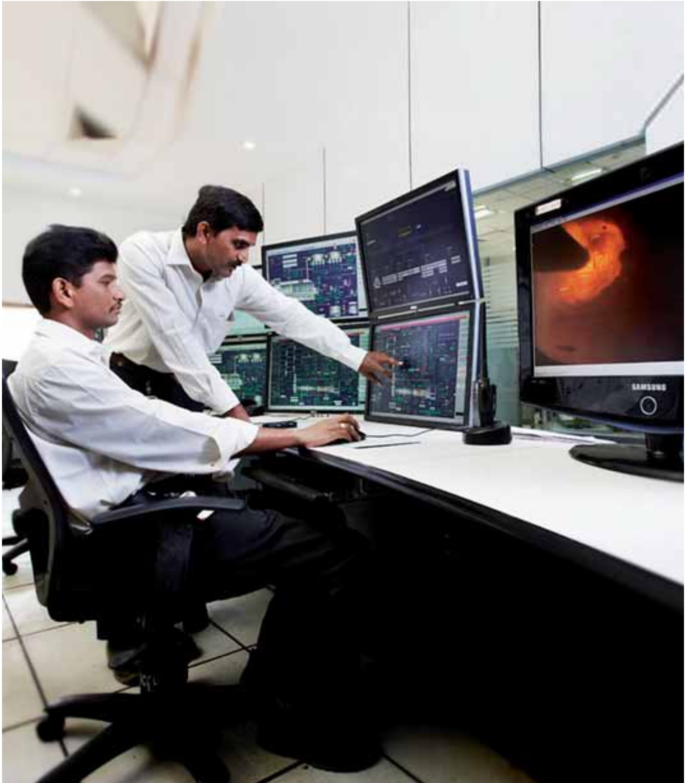
▲ The Bharathi Cement factory's control room (India).
