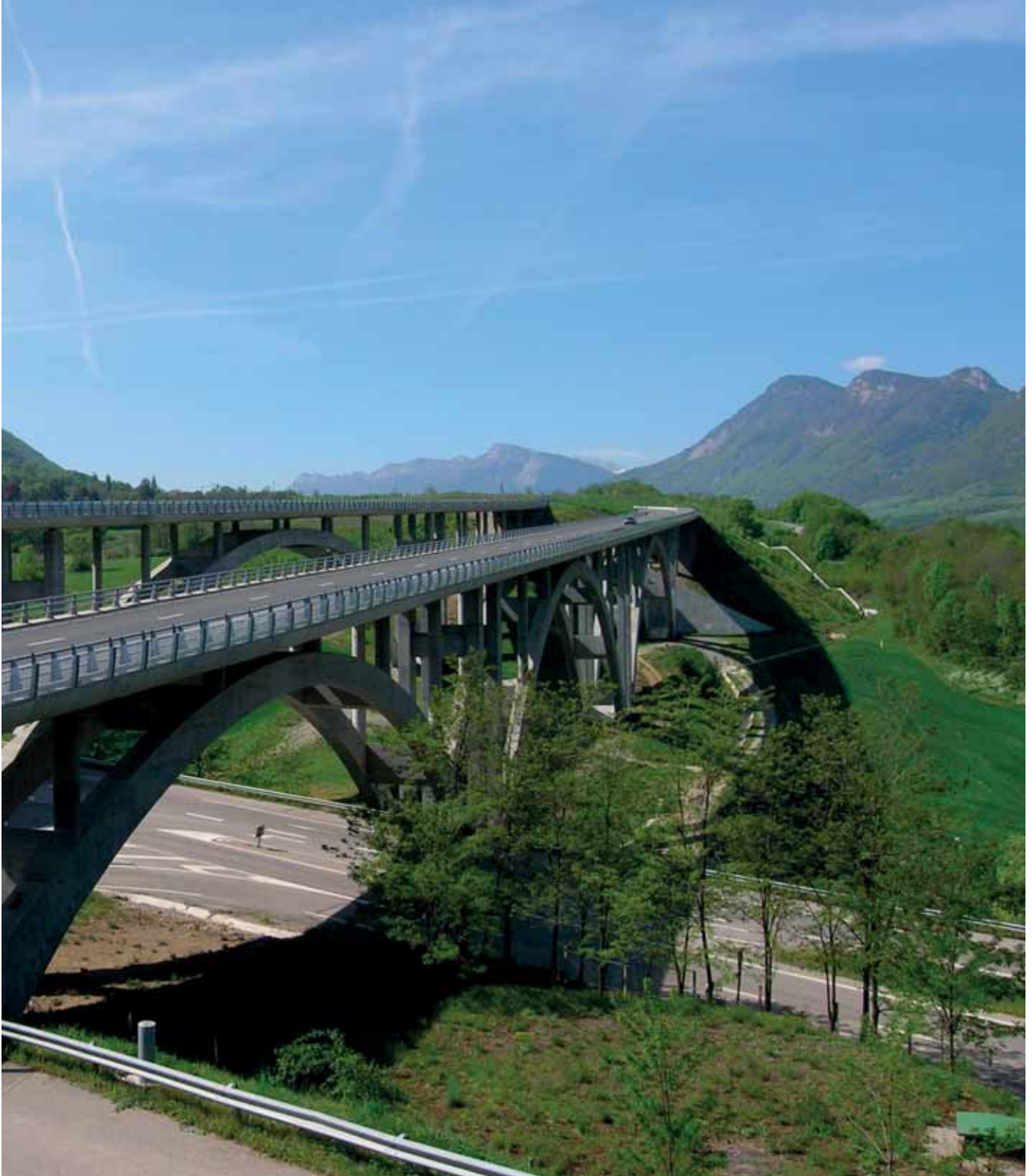
▲ The Crozet viaduct (France).
