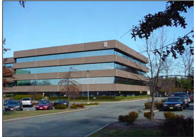
Existing Office Building on Executive Boulevard.
