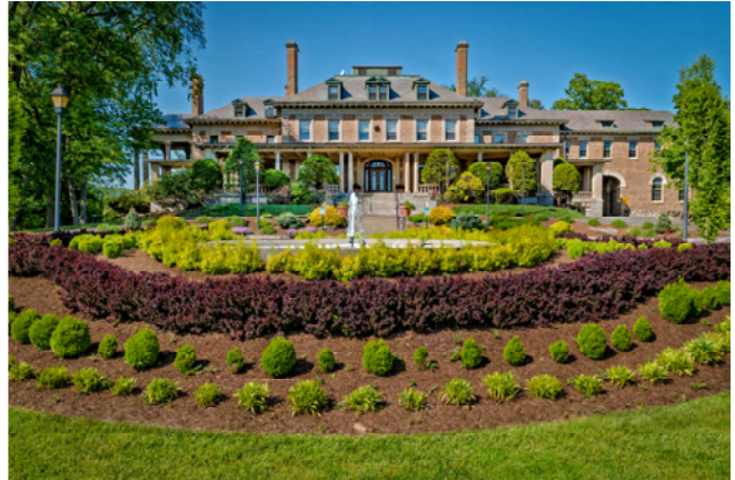
Existing mansion converted to offices
