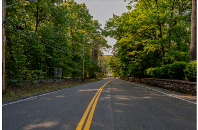
Montebello Road exhibits both traditional dry-laid stone farm walls (left) and mortared formal walls (right)
