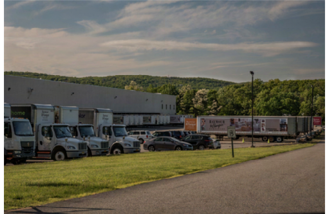
Warehouse and Distribution accessed via Dunnigan Drive
