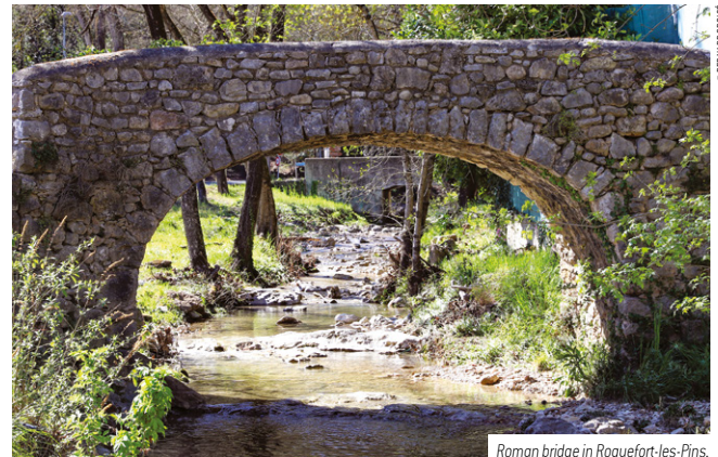
Roman bridge in Roquefort-les-Pins.
